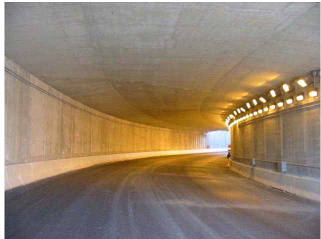
Figure 2 – Highway 404 HOV Tunnel
