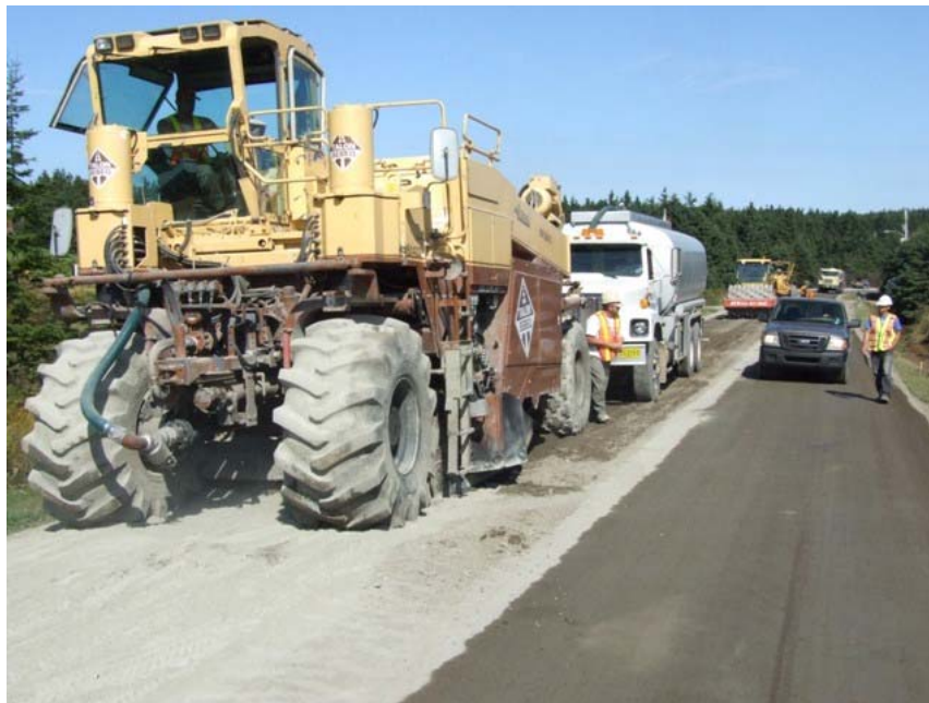
Figure 6 - Stabilization of the FDR.
