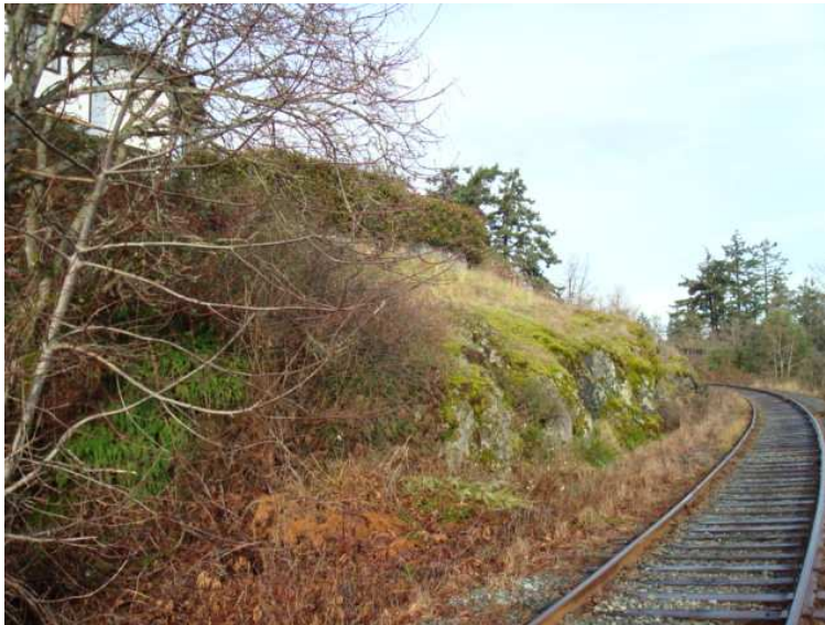
Photo 4 – Rock Excavation Area, View Royal, BC
