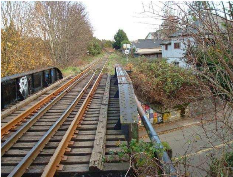
Photo 3 – Hereward Road Bridge, Victoria, BC
