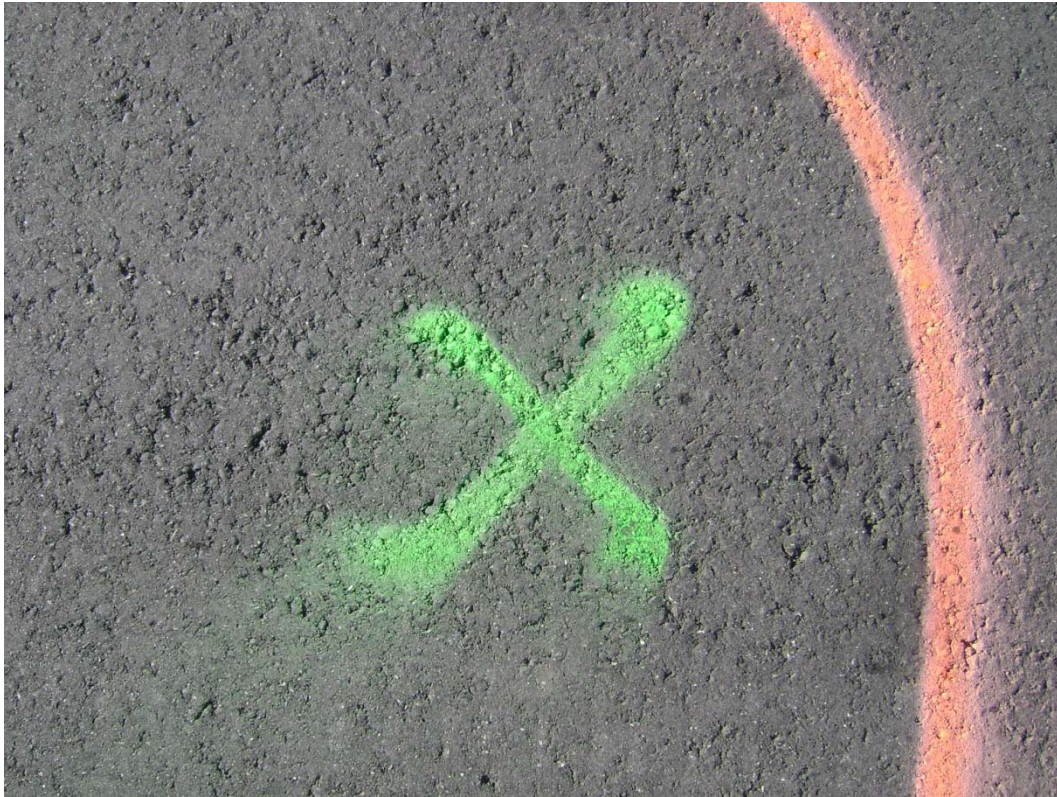
Figure 3 Localized segregated Asphalt Surface of Test Section
