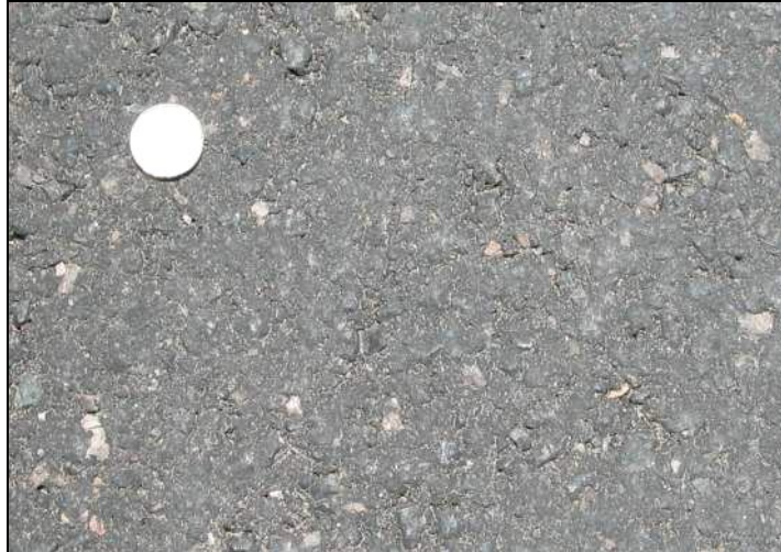
Figure 4. Surface Texture of CIR Mix
