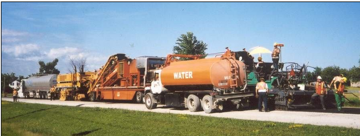
Figure 3. Cold-In-Place Recycling with Expanded Asphalt Train
