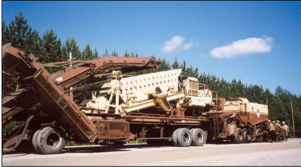
Figure 2. Cold-In-Place Recycling Train
