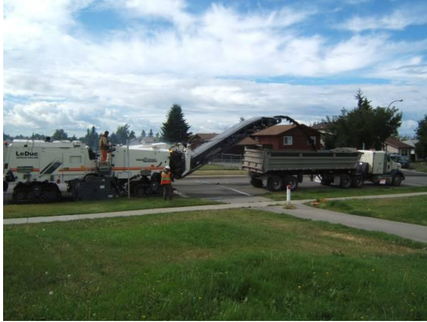
Roads crews in the midst of planing.
