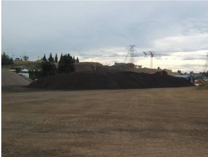
Stockpiling bulk aggregate.
