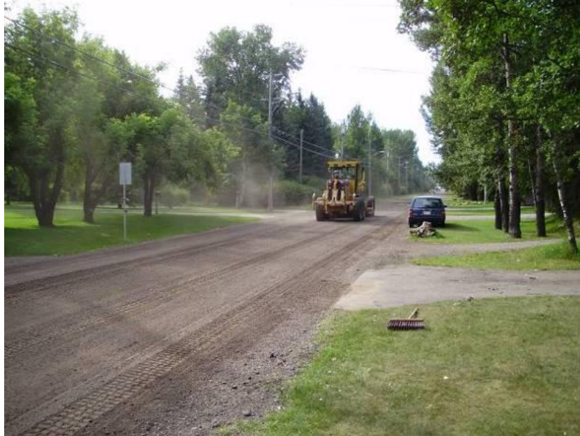
Roads crews scarifying a road.
