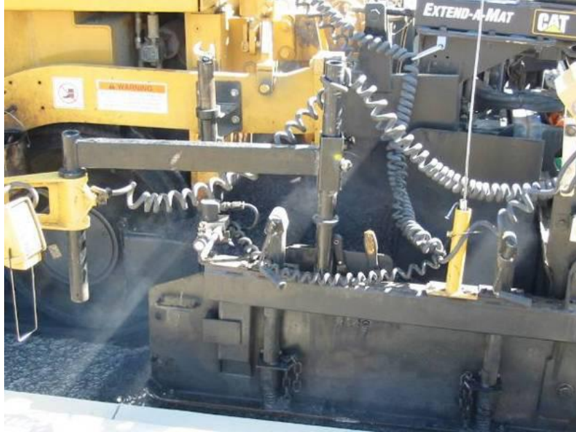
City crews paving.
