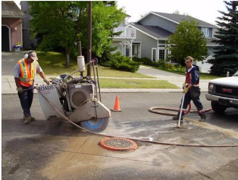
Roads crews saw cutting asphalt.
