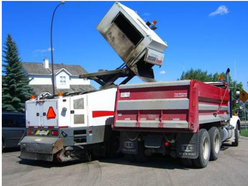
A Roads crew hauling milled asphalt.
