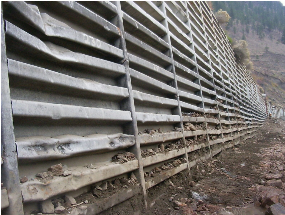
Photo 1: Typical Condition of the Bin Wall
