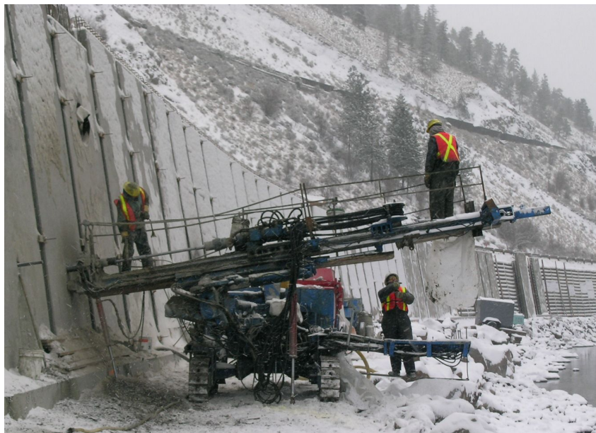
Photo 8: Drilling Anchors through the Wall
