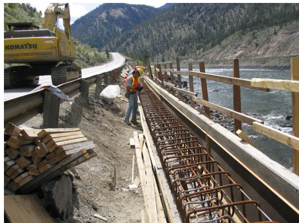
Photo 10: Cope Beam Formwork and Reinforcing
