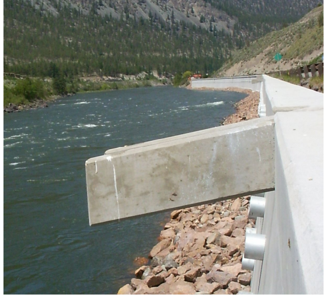
Photo 11: Precast Concrete Drainage Trough
