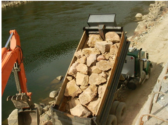
Photo 15: Riprap Installation in Progress
