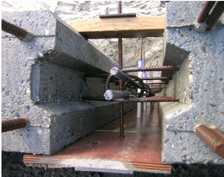
Photo 6: Top View of Shear Key
