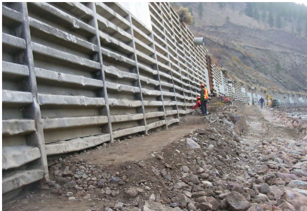
Photos 3 and 4: Ground Preparation and Footing Construction
