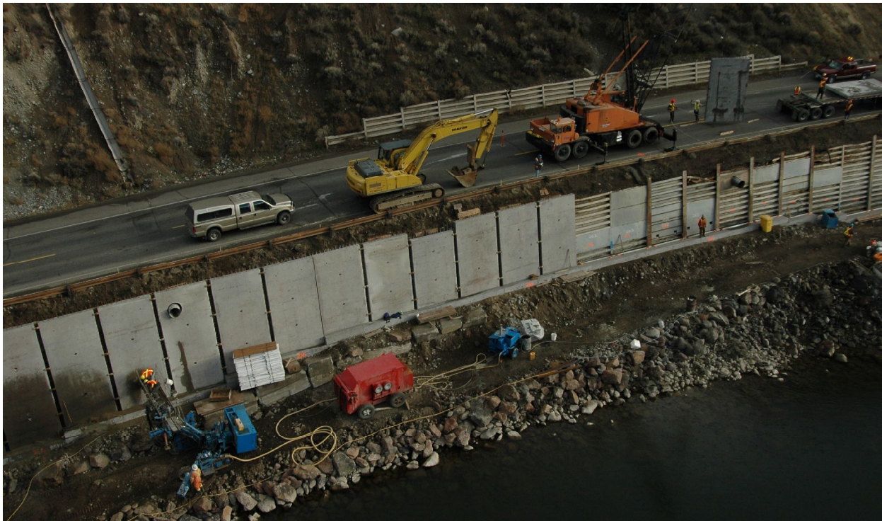
Photo 14: Aerial View of the Concrete Panel Installation Operations
