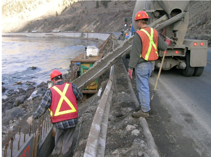
Photo 7: Placing Controlled Density Fill
