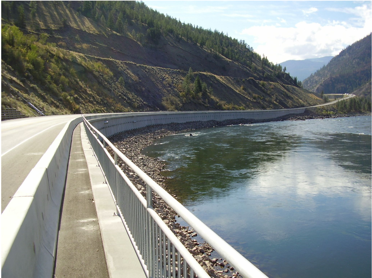
Photo 17: Completed Thompson River Retaining Wall Rehabilitation
