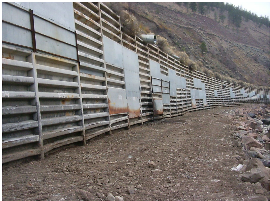
Photo 2: Typical Temporary Repairs to the Face of the Bin Wall
