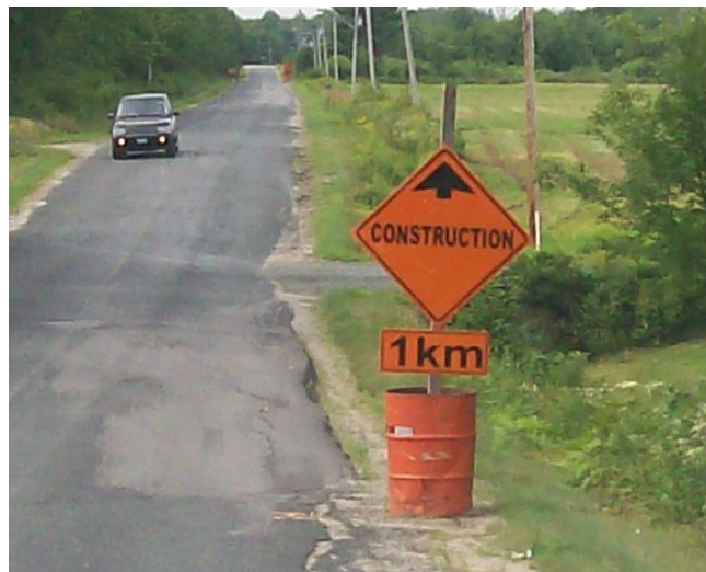
Figure I: Sign Mounted in Orange Steel Drum
