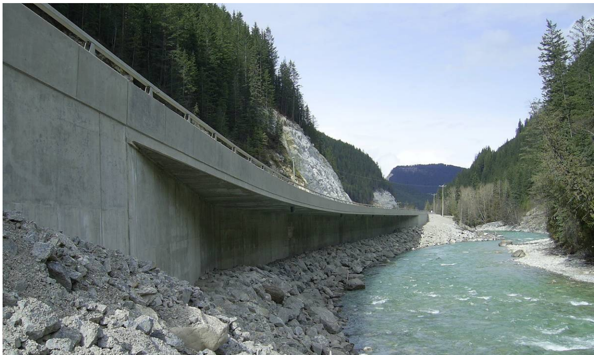
Picture 1 – Cantilever Structure
