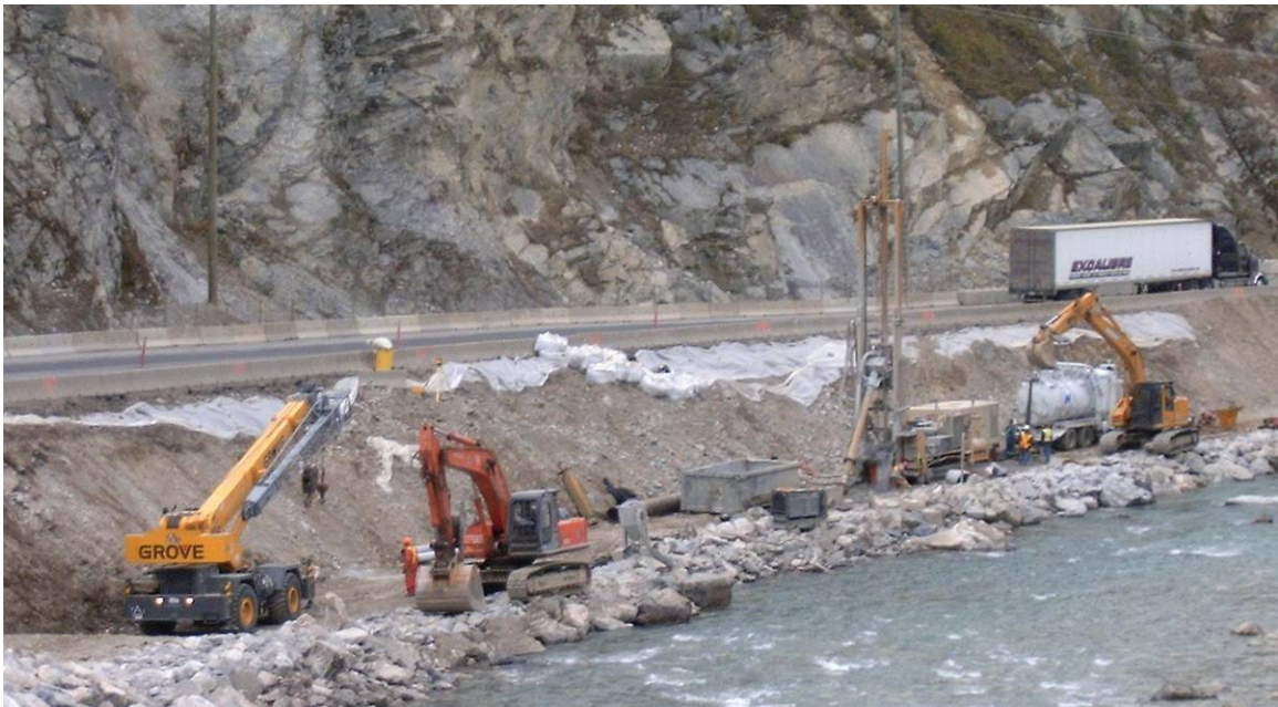
Picture 2 – Pile Installation
