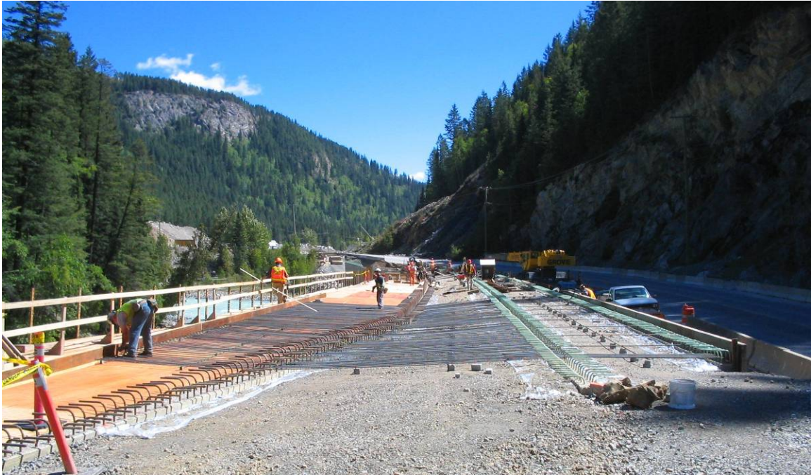
Picture 4 – Deck Construction
