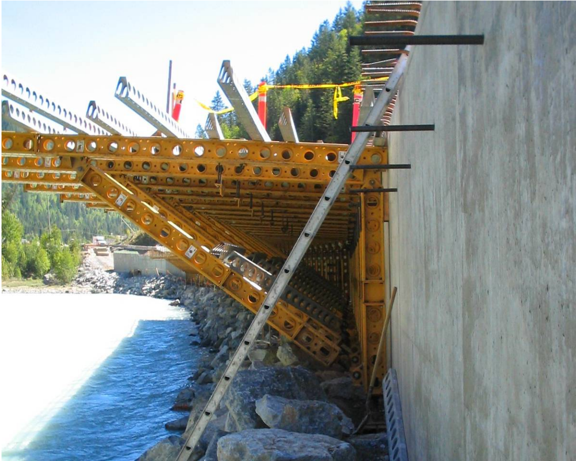
Picture 3 – Cantilever Formwork
