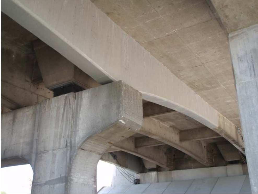
Figure 9 Queensborough Bridge - Fascia Girder Strengthening
