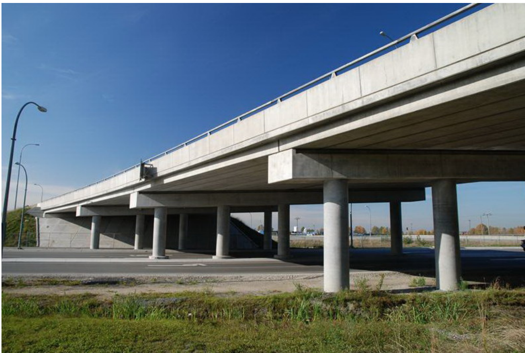
Figure 12 Completed Howes Overpass
