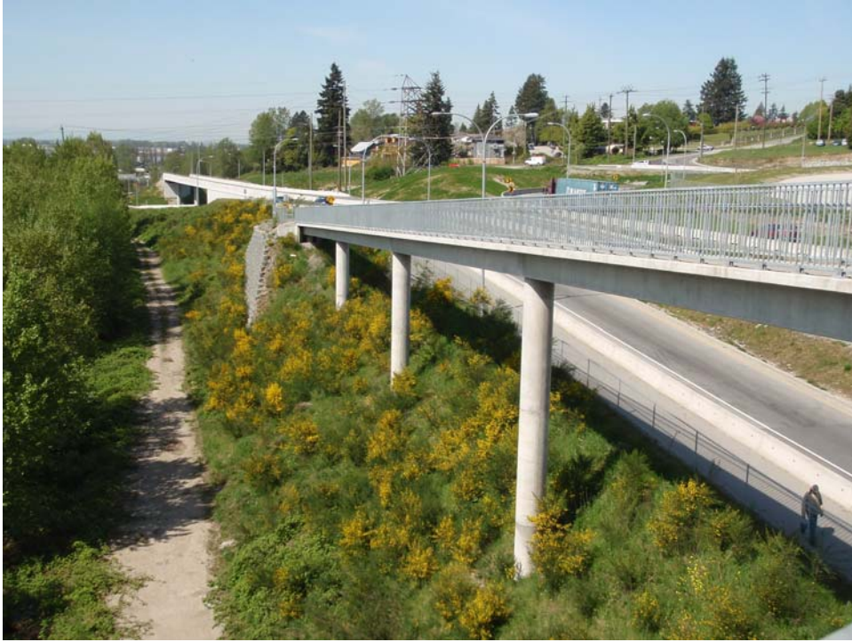
Figure 5 New Queensborough Bridge West Pedestrian Ramp
