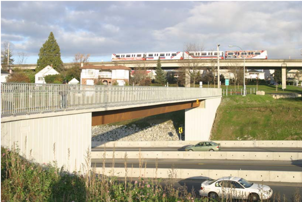
Figure 11 22nd Street Pedestrian Overpass
