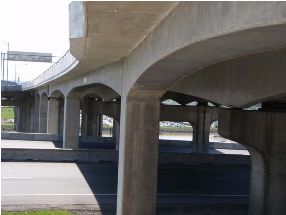
Figure 6 Queensborough Bridge North End Widening
