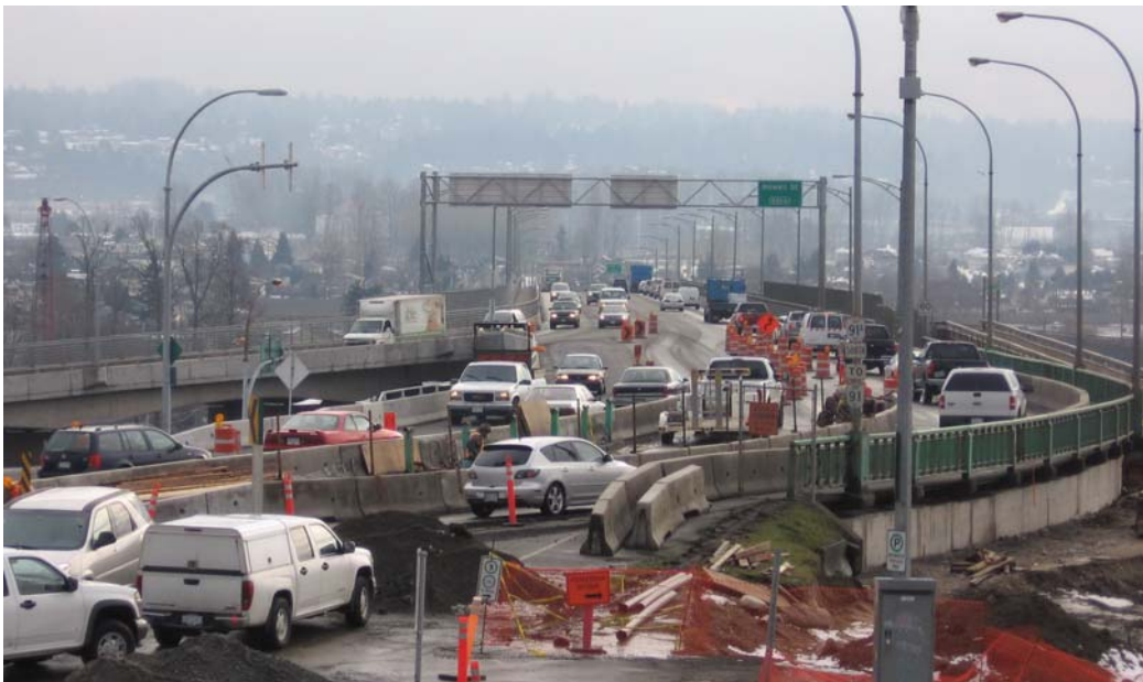
Figure 8 Queensborough Bridge - Traffic Detour for North End Span Removal
