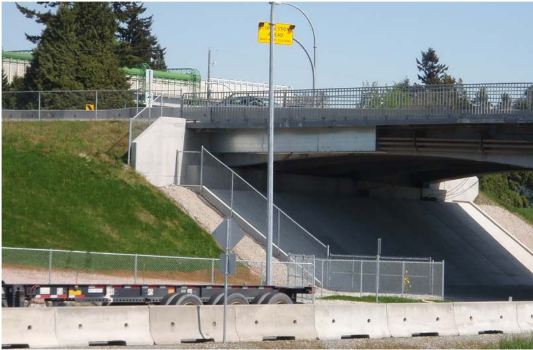
Figure 7 Queensborough Bridge's New North Abutment
