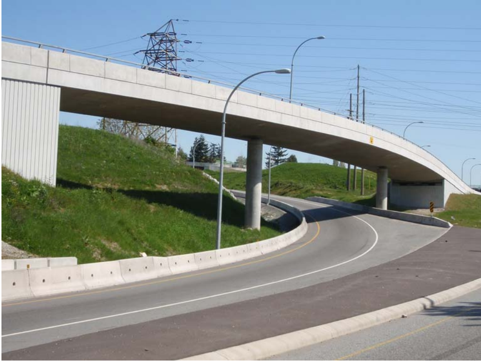
Figure 10 Completed Marine Way Flyover
