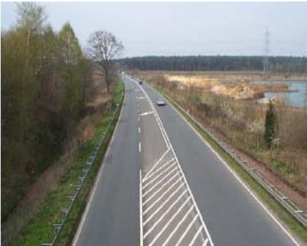
2+1 roadway in Germany
