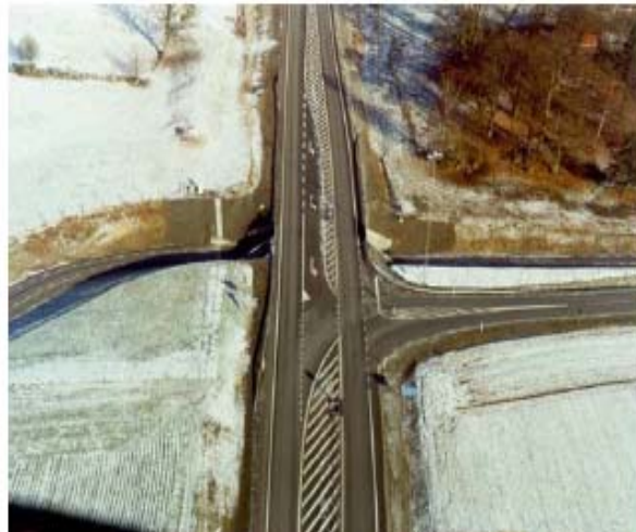
Three-legged intersection on 2+1 roadway in Sweden
