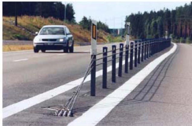
Cable barrier on a 2+1 road in Sweden
