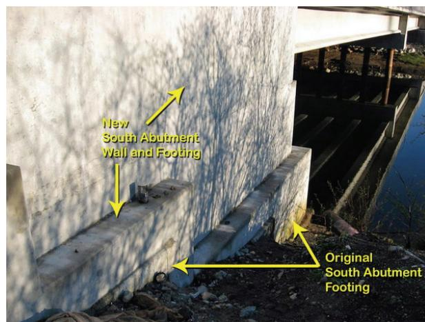
Figure 9 – Reuse of South Abutment Footing
