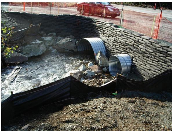
**Figure 27 - Deltalok Wall Before Vegetation (Dryden Creek Culvert, Inlet Headwall)**
