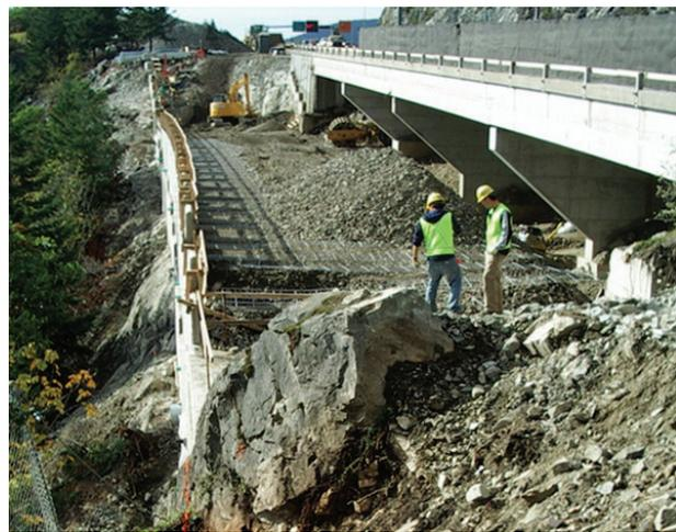
**Figure 24 - MSE Wall Construction (RW993)**
