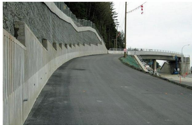
**Figure 26 - Tiered and Stacked Retaining Wall (RW87)**
