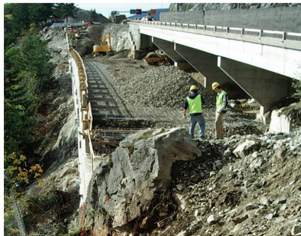
**Figure 24 - MSE Wall Construction (RW993)**
