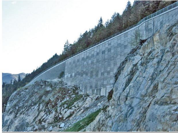
**Figure 23 - Completed Hybrid Retaining Wall (RW1025)**
