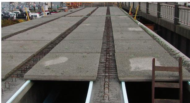
**Figure 6 – Precast Concrete Deck Panels**
