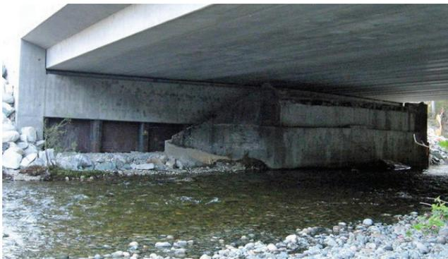
**Figure 16 – Retained North Abutment and Steel Scour Protection Plates**
