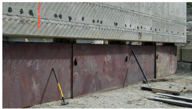
**Figure 17 – Backfill Side of Steel Scour Protection Plates**
