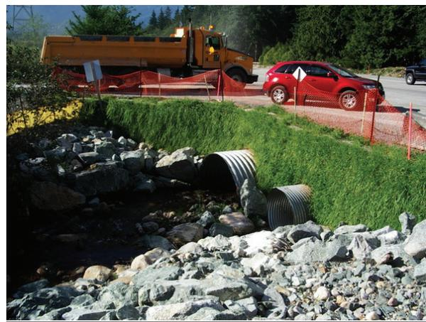
**Figure 28 - Deltalok Wall After Vegetation (Dryden Creek Culvert, Inlet Headwall)**
