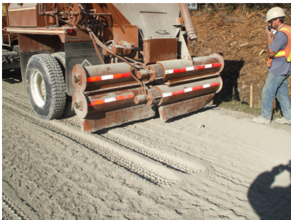
Figure 5 Dry cement application and mixing operations.
