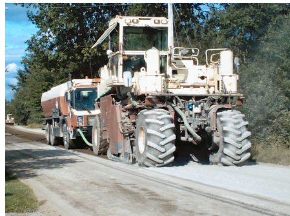
Figure 5 Dry cement application and mixing operations.
