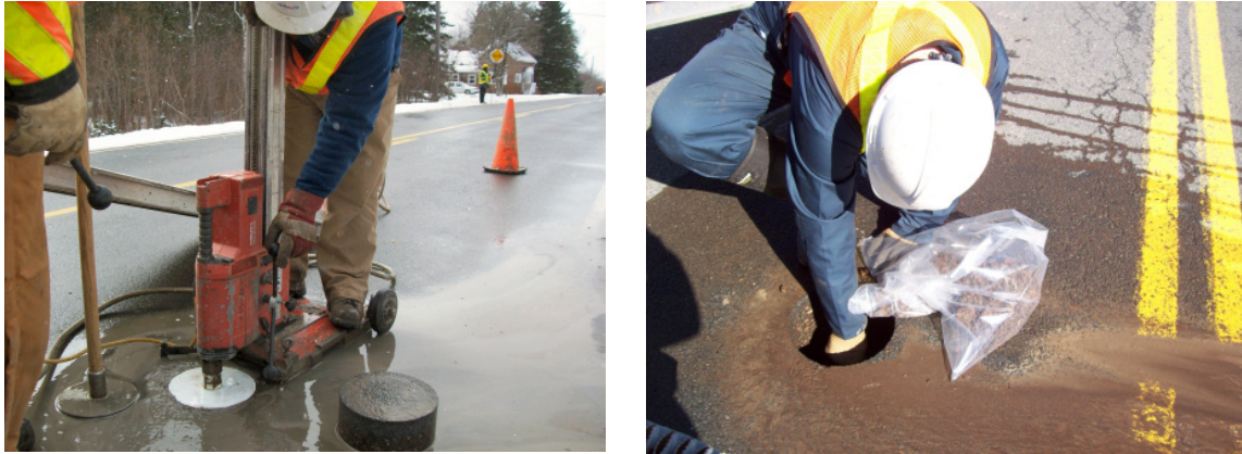
Figure 2 Large diameter coring and retrieval of underlying material.
