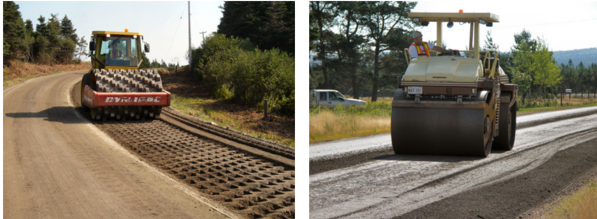
Figure 6 Pad foot (initial compaction) and final compaction operations.
