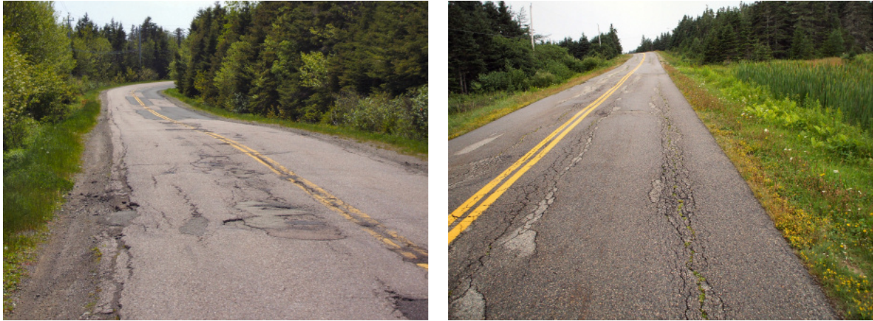
Figure 8 Pavement distresses at Main-a-Dieu and Point Michaud before FDR
