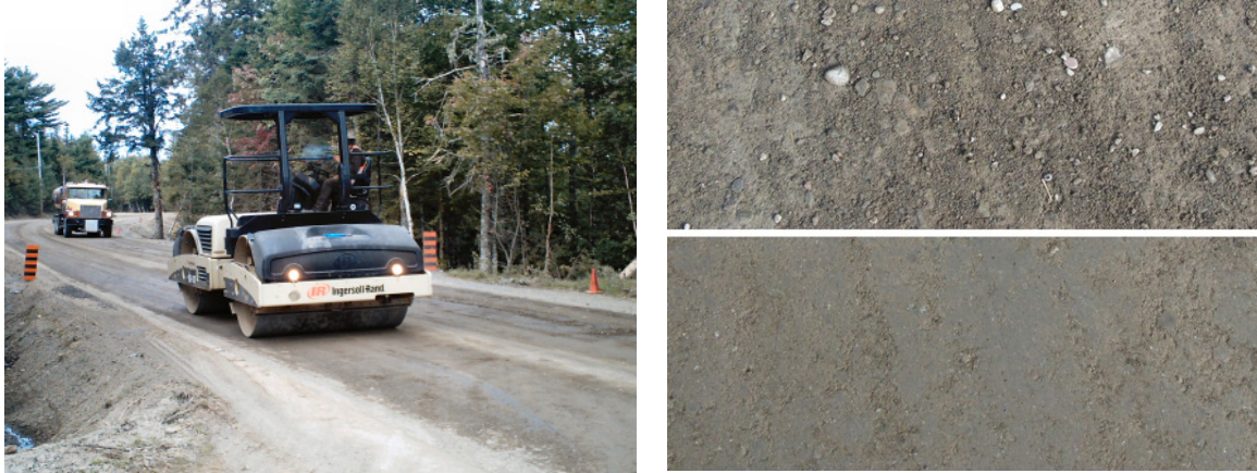
Figure 7 Inducing micro cracks and the treated material before and after rolling
