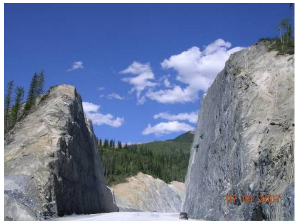
Photograph 2: 70m high through cut East of Bridge
