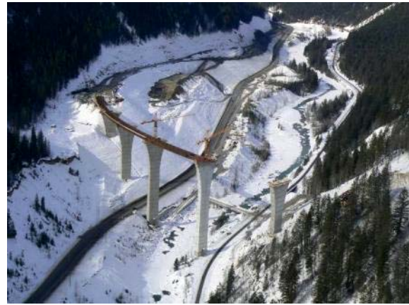
Photograph 5: Launching Bridge Beams
