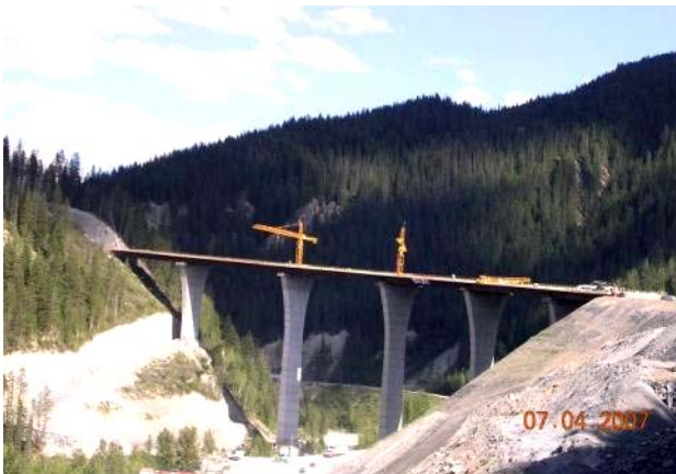
Photograph 4: New Park Bridge
