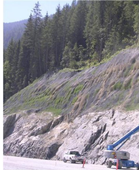
Photograph 3: West End Cuts in Quartzite with Tecco Mesh
