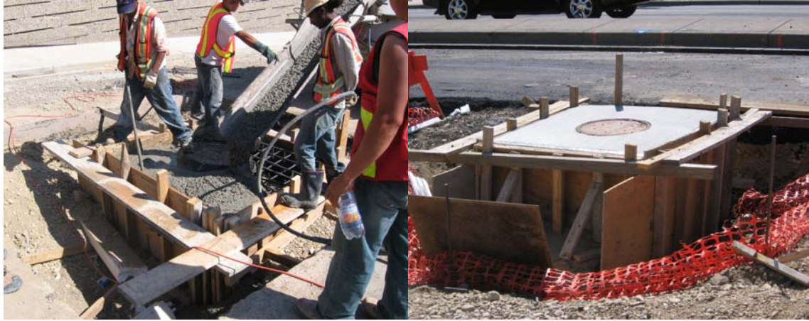
Figure 16: Installation of Cast-In-Place Manholes
