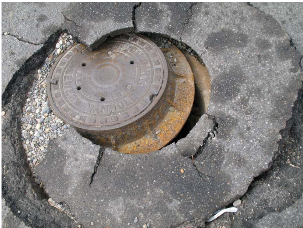
Figure 15: Primary Point of Failure at Storm Manhole
