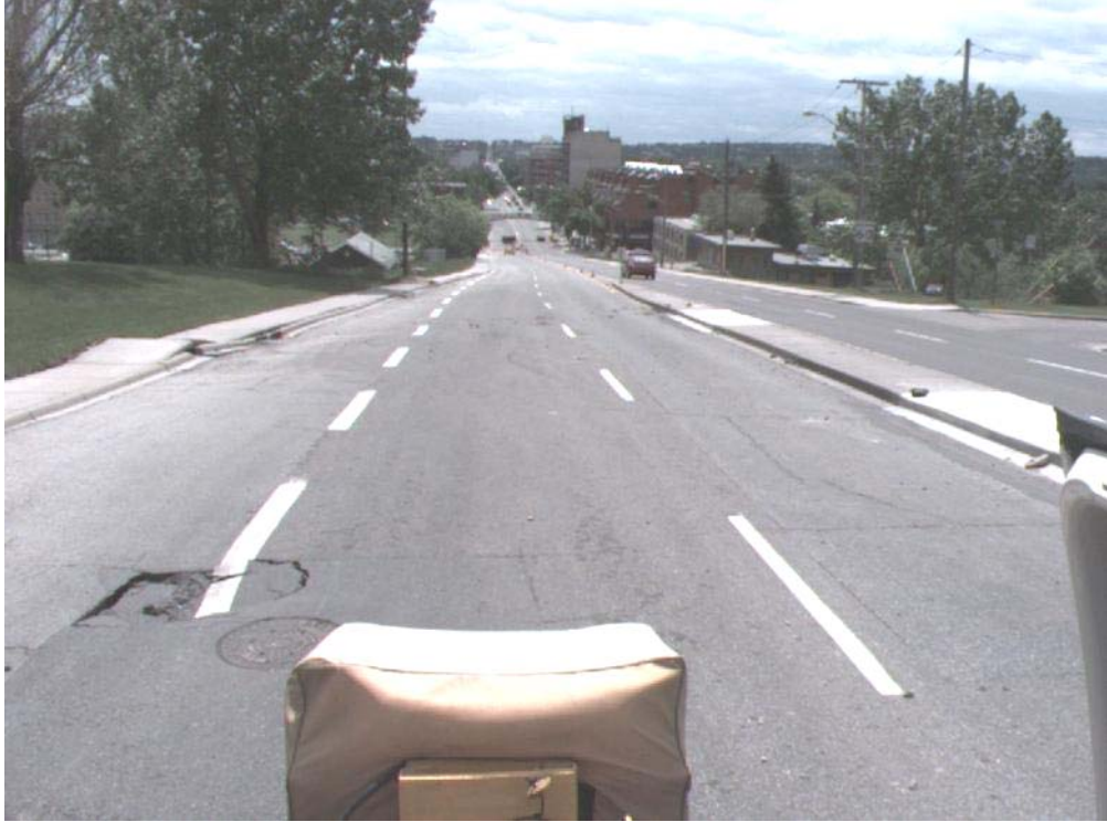
Figure 4: 14 Street NW Pavement Distress
