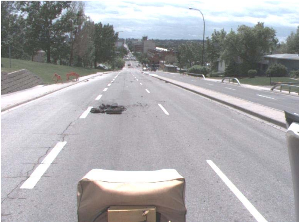
Figure 5: 14 Avenue NW Pavement Distress
