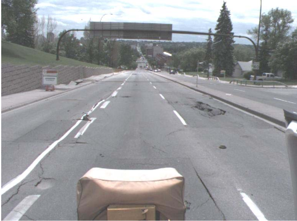
Figure 6: 14 Street NW Pavement Distress
