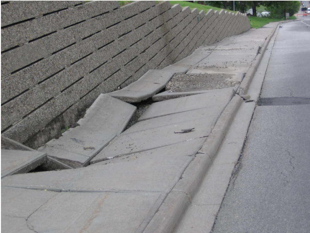
Figure 7: 14 Street NW Sidewalk Distress
