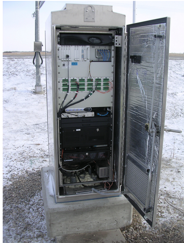
Figure 6 - Virtual Weigh Station Enclosure and Electronics Rack
