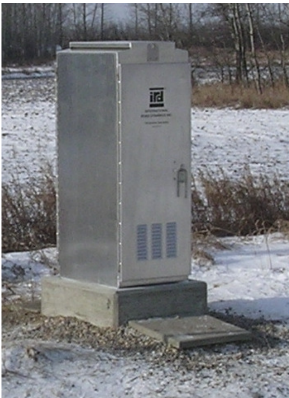
Figure 6 - Virtual Weigh Station Enclosure and Electronics Rack
