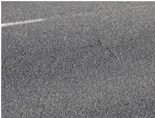
Photo 6: Alligator Failure North Bound Slow Lane
