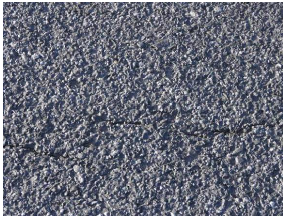
Photo 1: Driving Lanes Phase 1 - 200 m from South End – Note Structural Cracking
