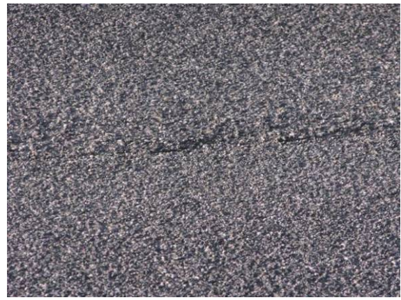
Photo 3: Longitudinal Joint Failure - Same Area as Photo 1 and 2
