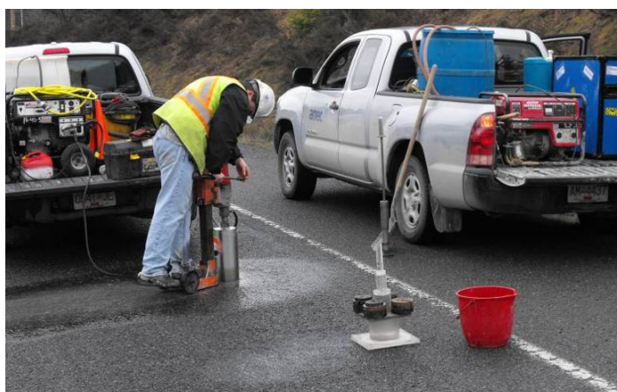
Photo 14: Coring and Permeability Testing
