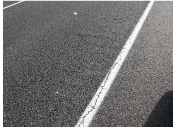
Photo 5: Alligator Fatigue Cracking about 400 m North of Project Start
