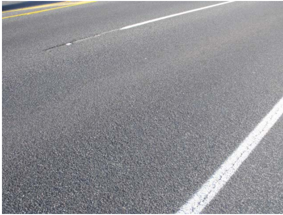
Photo 4: Wheelpath Wear Phase 1
