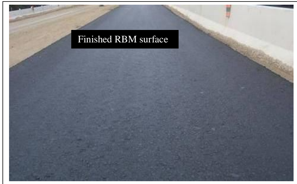
Figure 3 Rich bottom mix placed on Hwy 401
