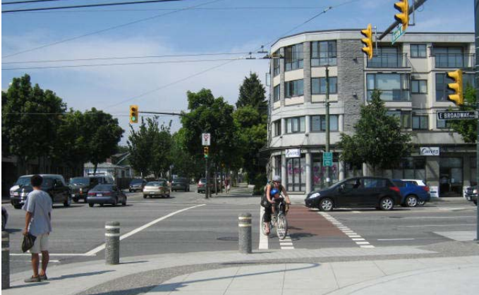
Figure XII - Separated Cross-Bike at Grandview Highway North and Victoria Drive
