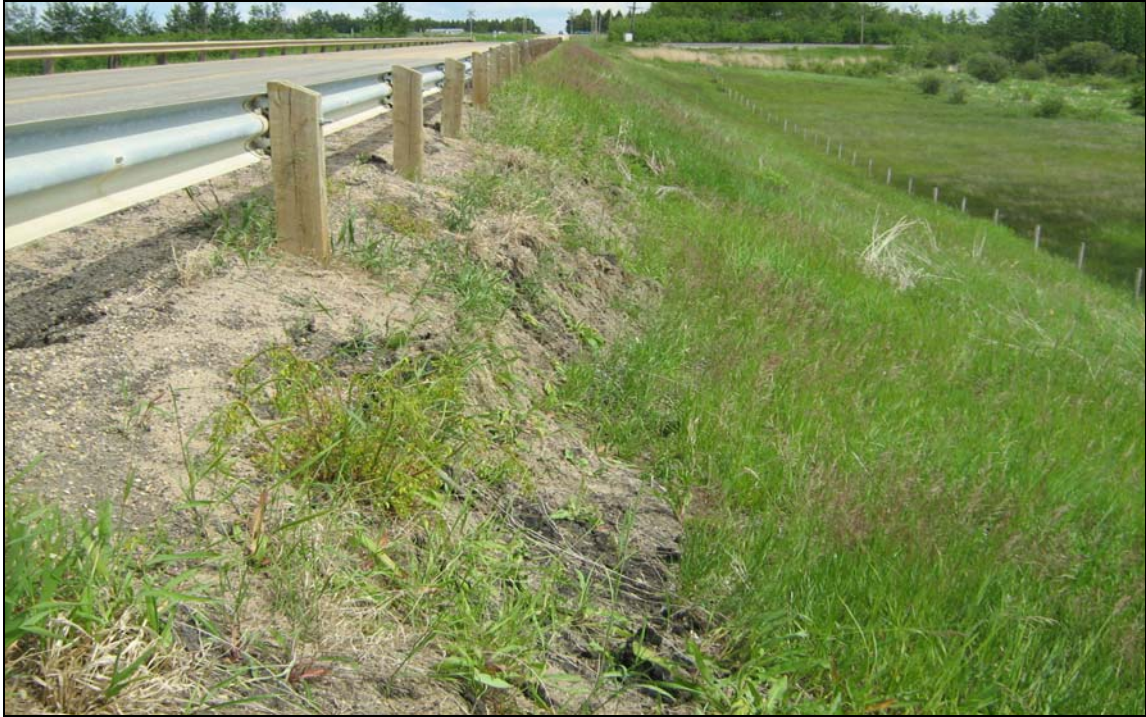
PHOTO 2: Looking eastbound; notice the vertical scarp close to the guardrail posts
