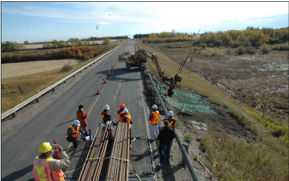
PHOTO 3: Advantage of using soil nailing is that only a single lane closure is needed and this reduces road user disruptions
