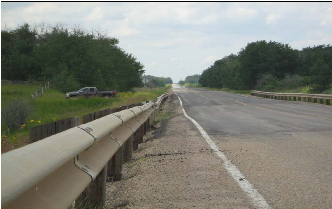
PHOTO 1: Looking west along the eastbound lane; notice the sag in the guardrail & roadway
