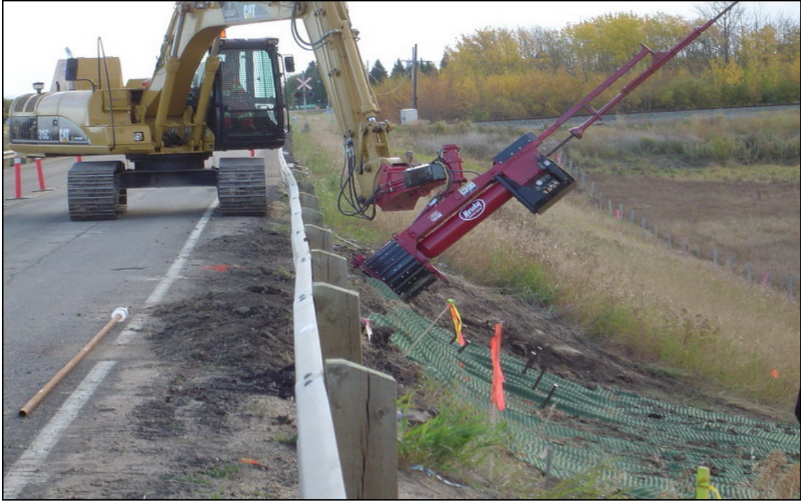
PHOTO 4: Closer look at the launcher's ability to reach around obstacles and utility services to install nails
