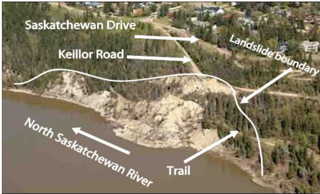
Figure 1 Keillor Road landslide (May 2005, the City of Edmonton)
