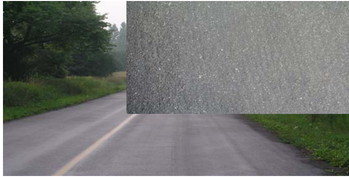
Figure 3 – Cape seal applied on Halls Road in Whitby, Ontario
