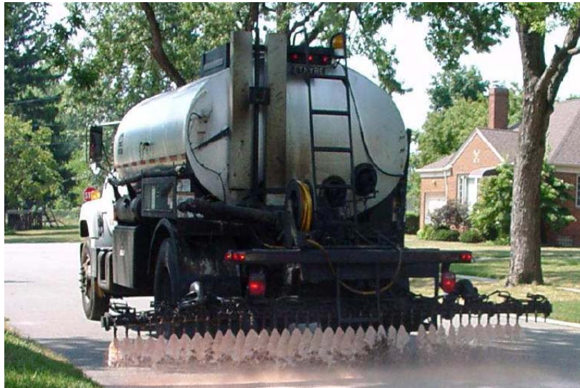
Photograph 1 Application of Reclamite on asphalt pavement [PTI].
