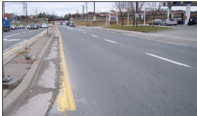
Photographs 4 Condition of micro-surfacing on Thicksen Road in Whitby 11 years after application
