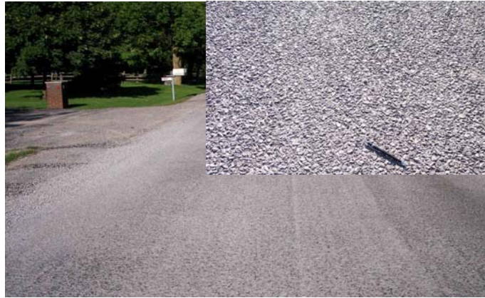
Photograph 2 Chip seal applied on Coates Road in Oshawa, Ontario
