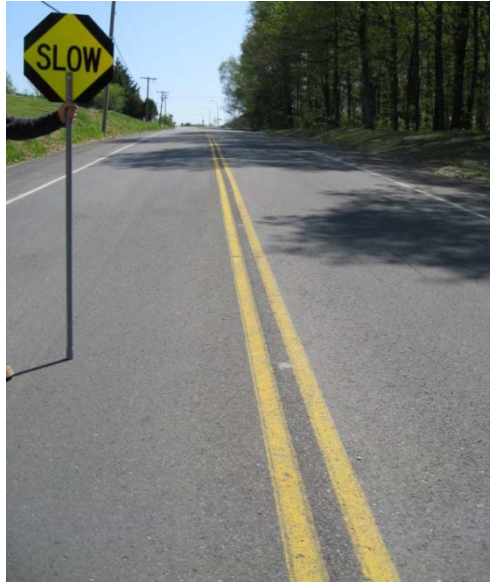
Photograph 9 Pavement condition near the centreline of Jerseyville Rd paved with joint heaters.
