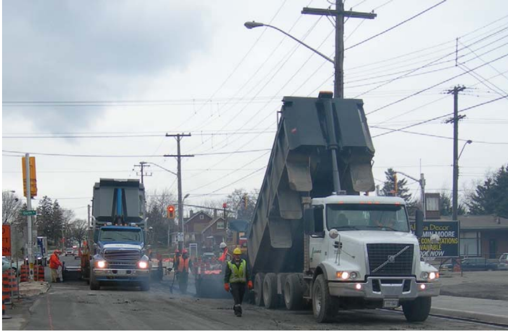
Photograph 1 Echelon paving on Garth Street in Hamilton in 2008.
