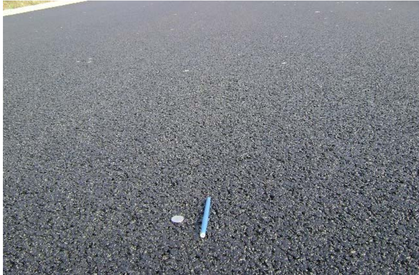
Photograph 6 Stone Mastic Asphalt surface course placed on the Red Hill Valley Parkway in Hamilton using echelon paving with MTV in 2007.
