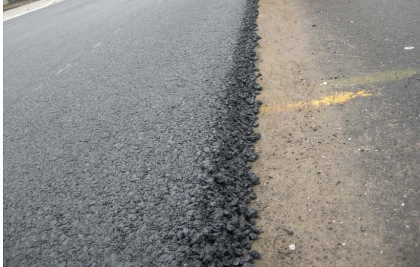
Photograph 4 Low density area in cold longitudinal joint.
