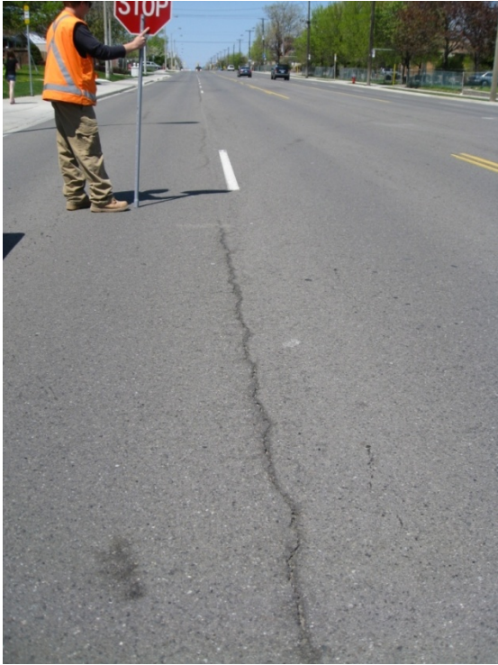
Photograph 12 Pavement condition at centreline of Mohawk Road paved with cold joints.
