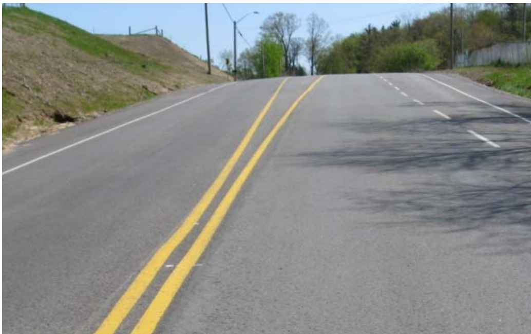
Photograph 5 Pavement condition of Jerseyville Road paved in echelon in 2007.
