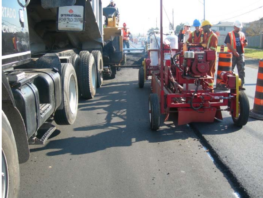
Photograph 8 Placement of Superpave 12.5 FC2 surface course using infrared joint heater on Rymal Road in Hamilton in 2008.
