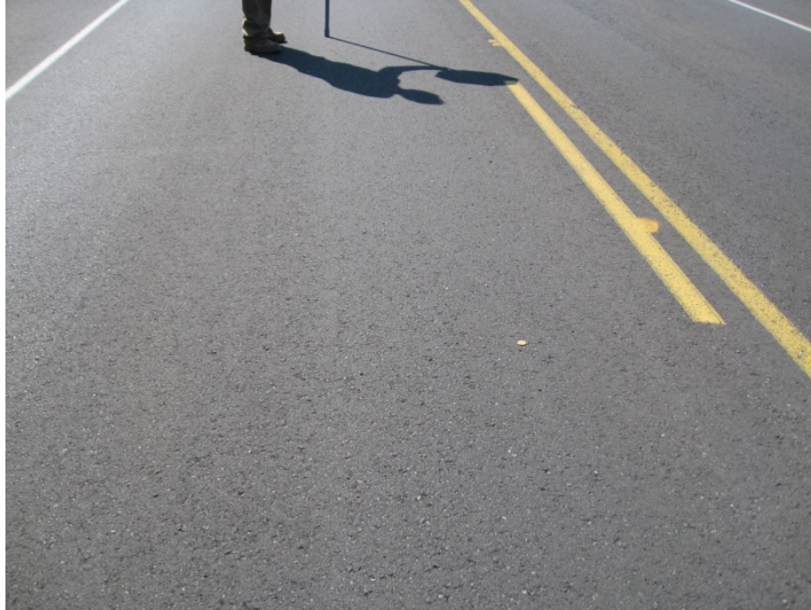
Photograph 7 Pavement condition of Sawmill Road paved in echelon with an MTV in 2007.
