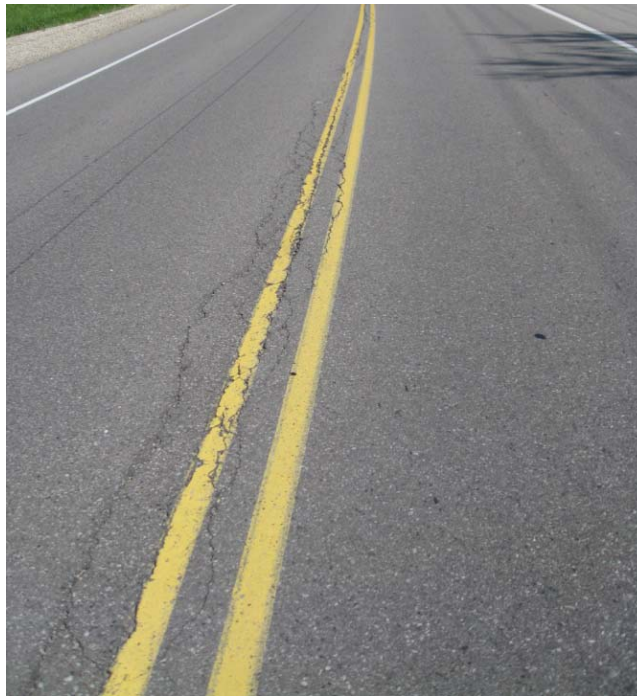
Photograph 11 Pavement condition at centreline of Sawmill Road paved with cold joints.
