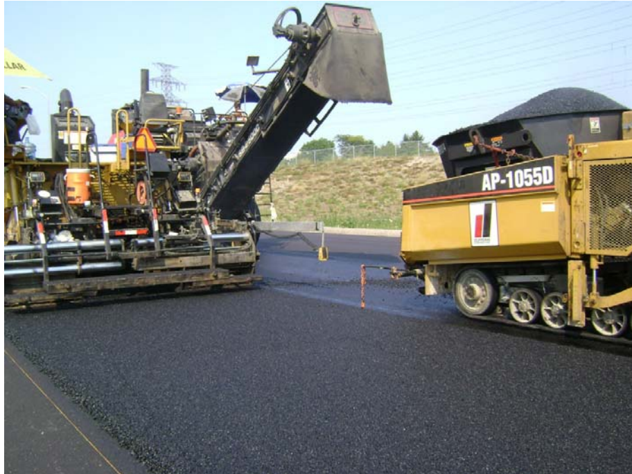
Photograph 2 Echelon paving with Shuttle Buggy ® MTV on the RHVP in Hamilton in 2007.
