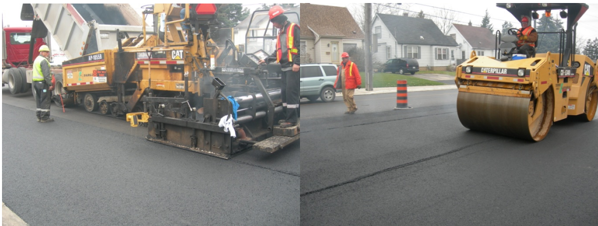
Photograph 10 Placement of warm mix asphalt Superpave 12.5 FC2 surface course and hot joint compaction on Garth Street in Hamilton in 2008.
