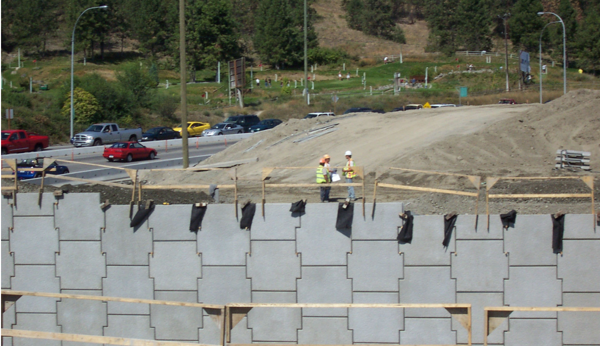
Figure 6. Constructing the MSE walls
