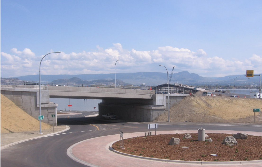
Figure 9. Campbell Road Overpass with South Roundabout
