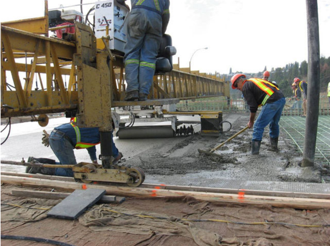
Figure 8. Pouring the concrete deck with Gomaco machine
