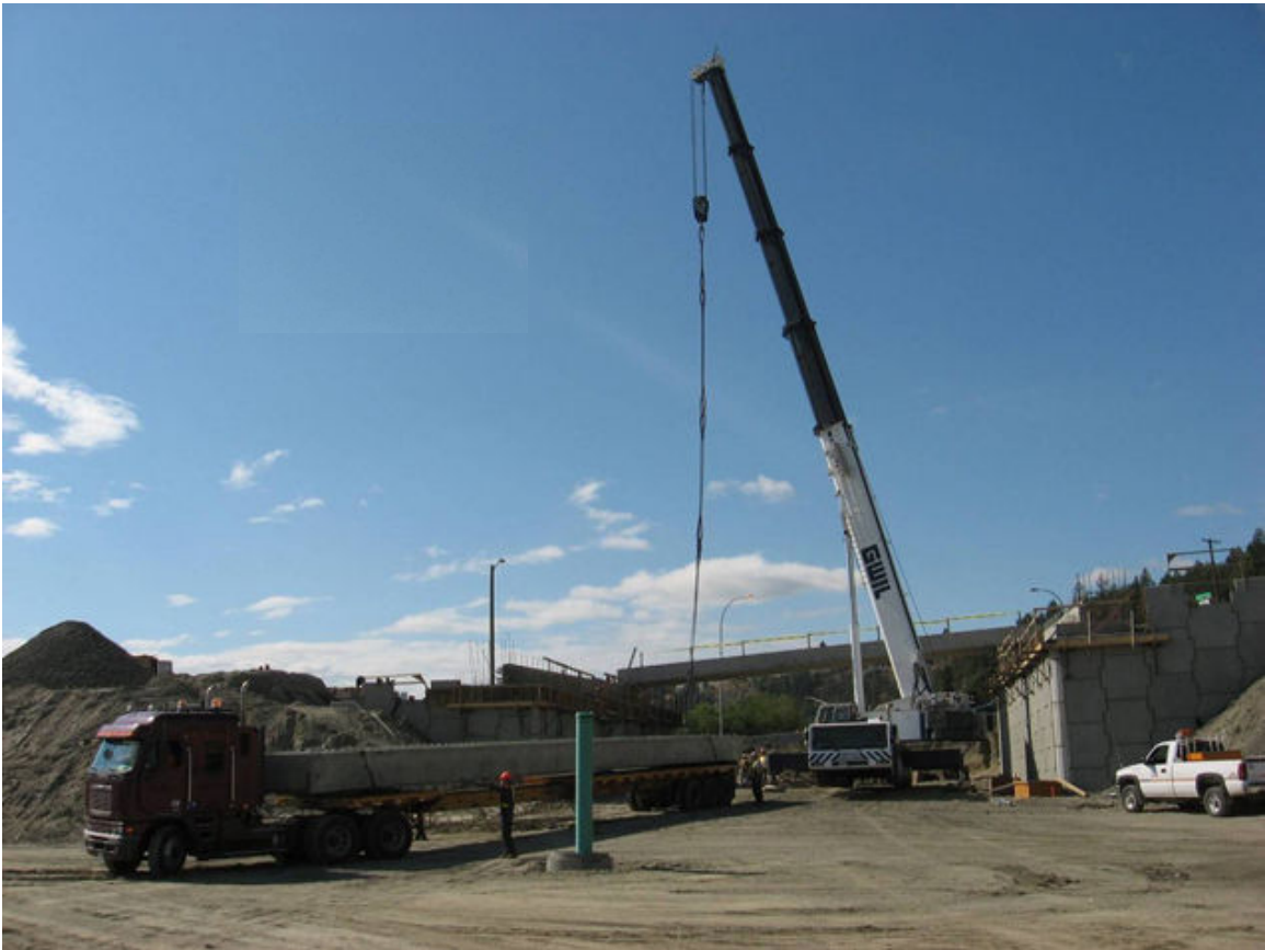
Figure 7. Erecting the precast box girders
