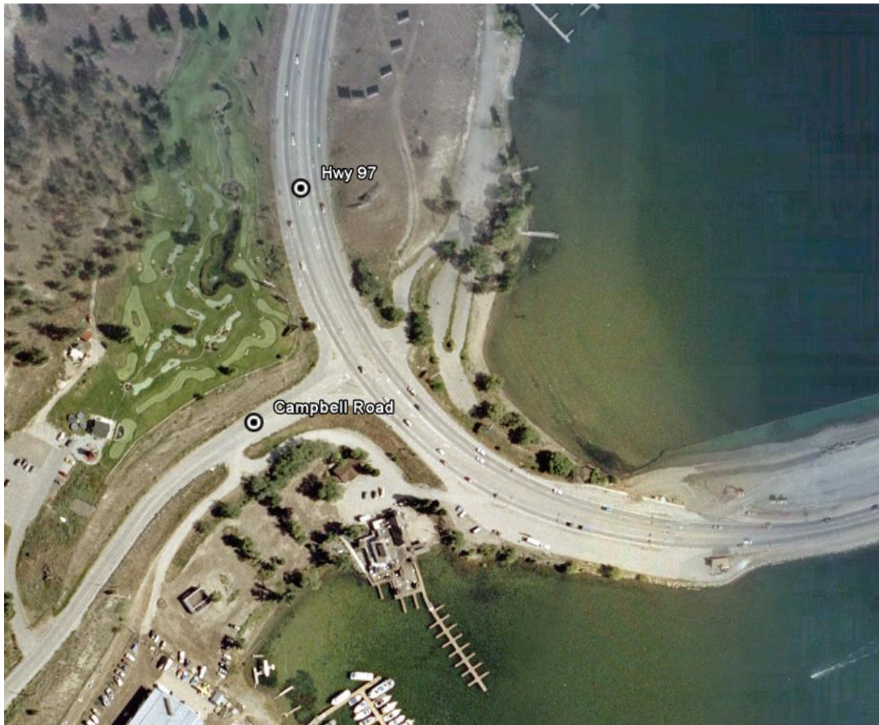
Figure 1. Aerial view of Campbell Road intersection before the overpass structure is built
