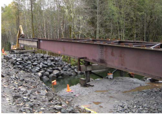
Figure 8 Typical Girder Launch
