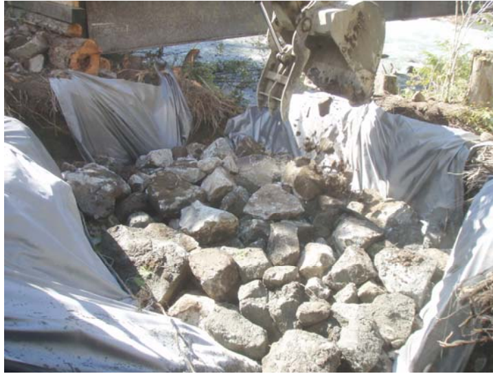
Figure 2 Rock fill enclosed in geotextile fabric
