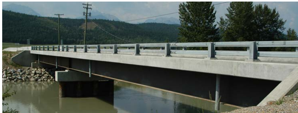
Figure 7 Top Mounted PL-2 Bridge Rail (posts at 3.048 m centres)
