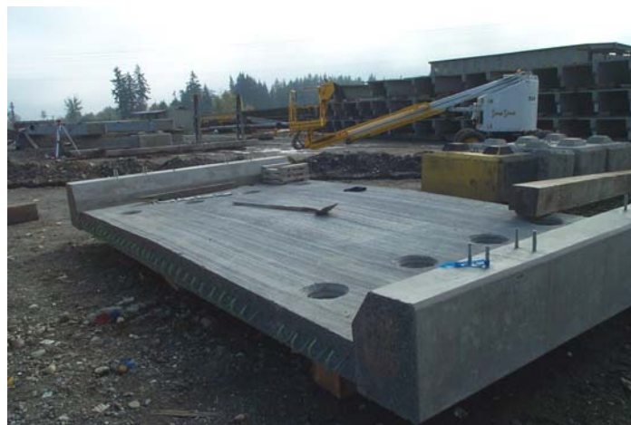
Figure 4 Typical Precast Concrete Deck Panel
