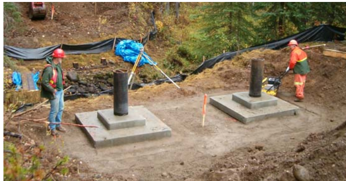
Figure 1 Installation of precast concrete footing
