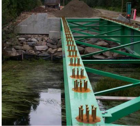
Figure 3 Typical Twin-Steel I-Girder and Precast Concrete Ballast Wall
