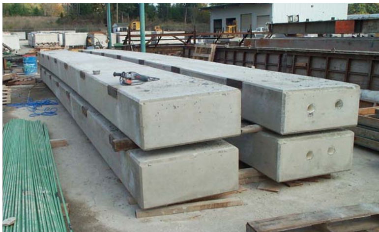
Figure 5 Welded Shear Connected Slab Girders
