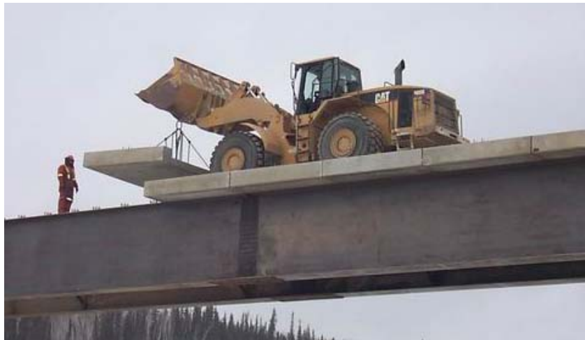
Figure 9 Placement of Precast Concrete Deck Panels
