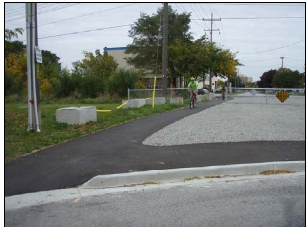
Good local street – trail connection
