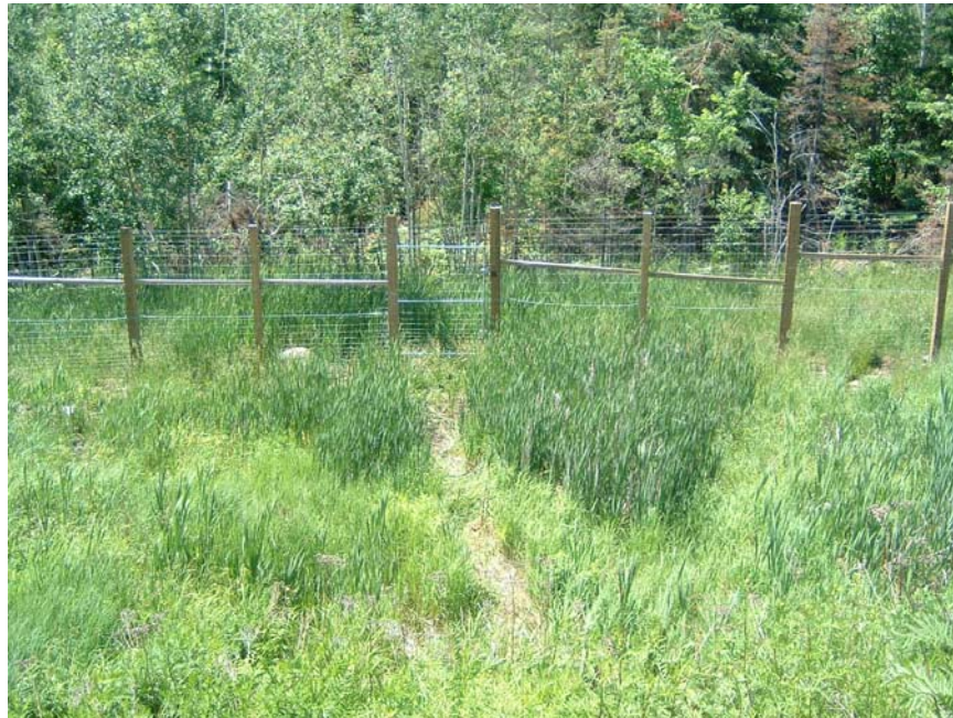
Figure 7. 2.8m Highway wildlife fencing, Highway 11 South of North Bay, one-way gate shown
