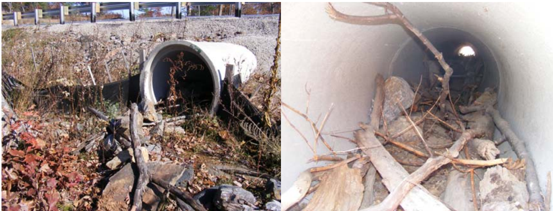
Figure 4. Herpetofauna culvert, dump road off of Highway 400, located in Eastern Massassauga Rattlesnake habitat
