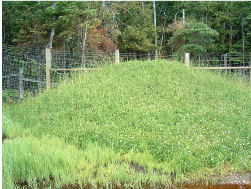
Figure 8. Figure 7. 2.8m Highway wildlife fencing, Highway 11 South of North Bay, jump-out ramp shown
