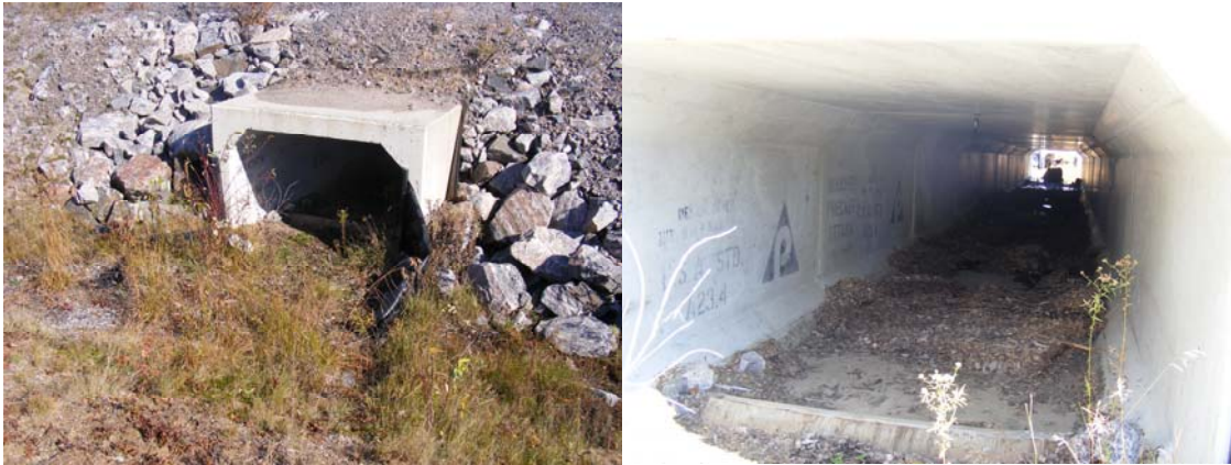
Figure 3. Herpetofauna culvert, Highway 400, North of Tower Road, located in Eastern Massassauga Rattlesnake habitat
