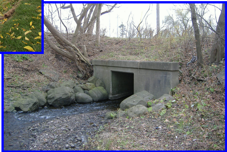
Photo 5: Existing Deficient Coronation Blvd. Culvert.
