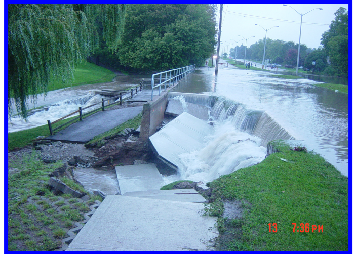
Photo 1: Coronation Blvd. in the City of Cambridge in 2005 Photo 2: Overtopping of “repaired” Coronation Blvd in 2006
