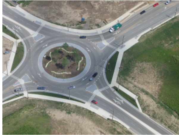
Photo: Ourston Roundabouts Canada
