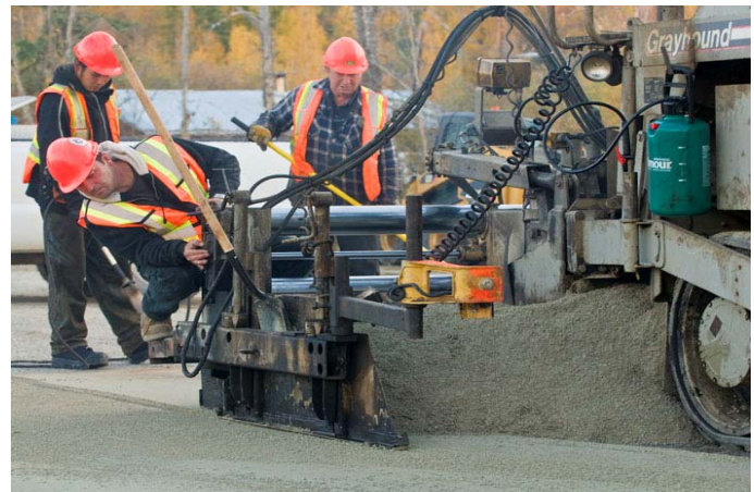
Figure 9 - Top layer of light coloured pavement
