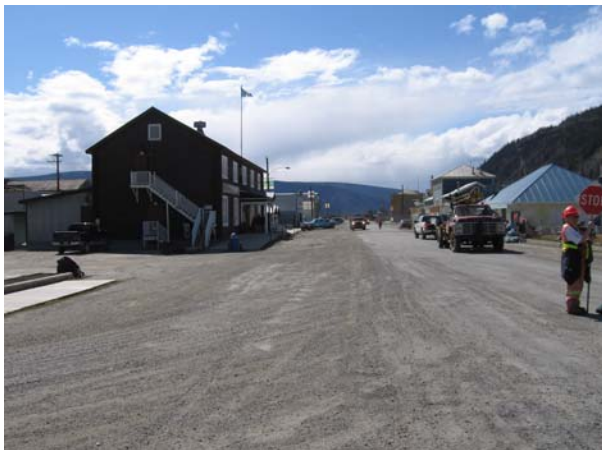
Figure 2 - Spring 2009, typical drainage problems and surface distresses along Front Street were a cause of community dissatisfaction
