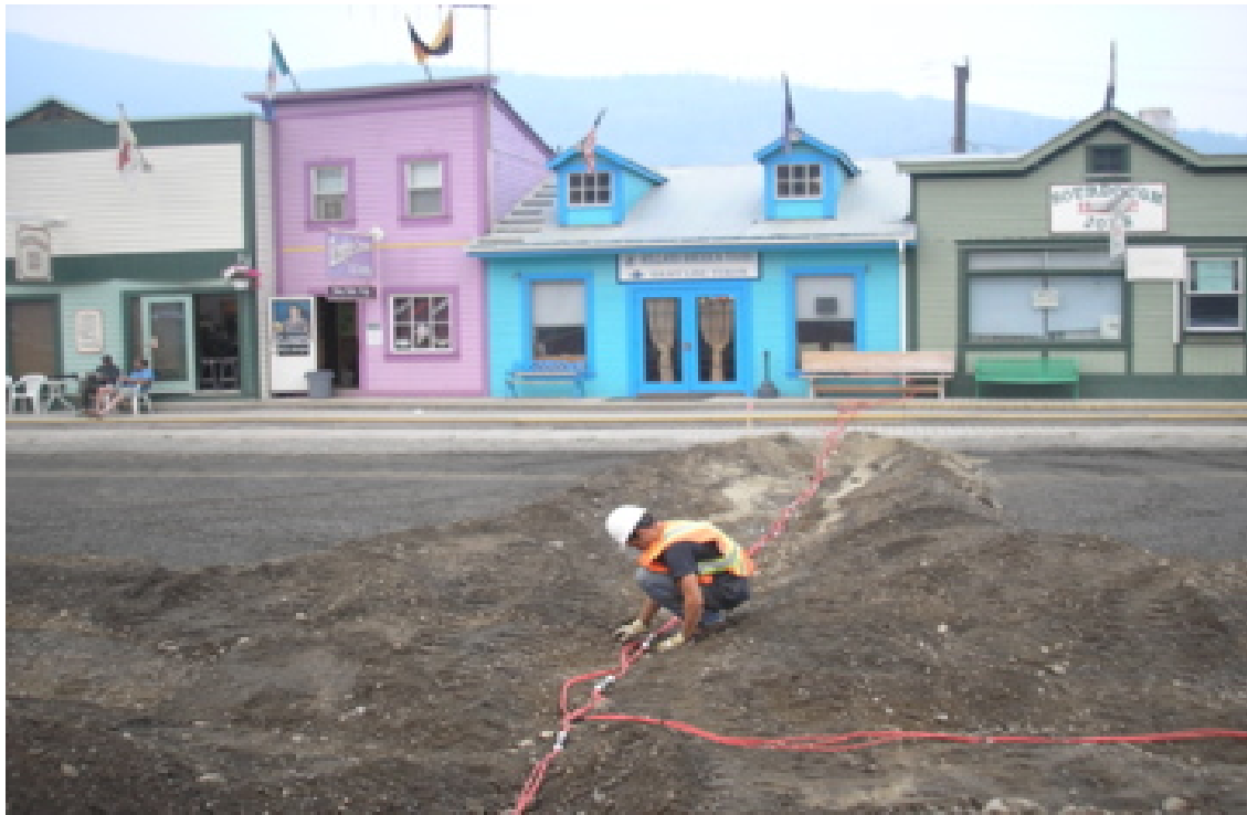
Figure 11. Installing DC Resistivity Array
