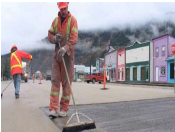
Figure 9 - Top layer of light coloured pavement
