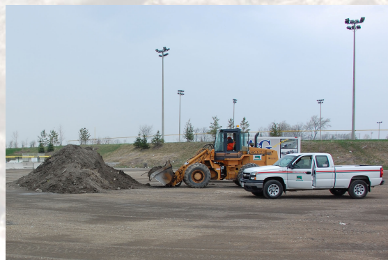
Figure 9. Removing sediment deposited on the asphalt pad after the snowpack melted.
