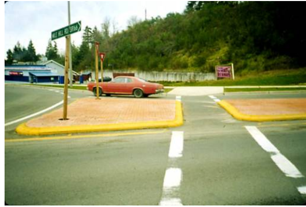
Figure 9 - Poor Crosswalk Layout and Alignment
