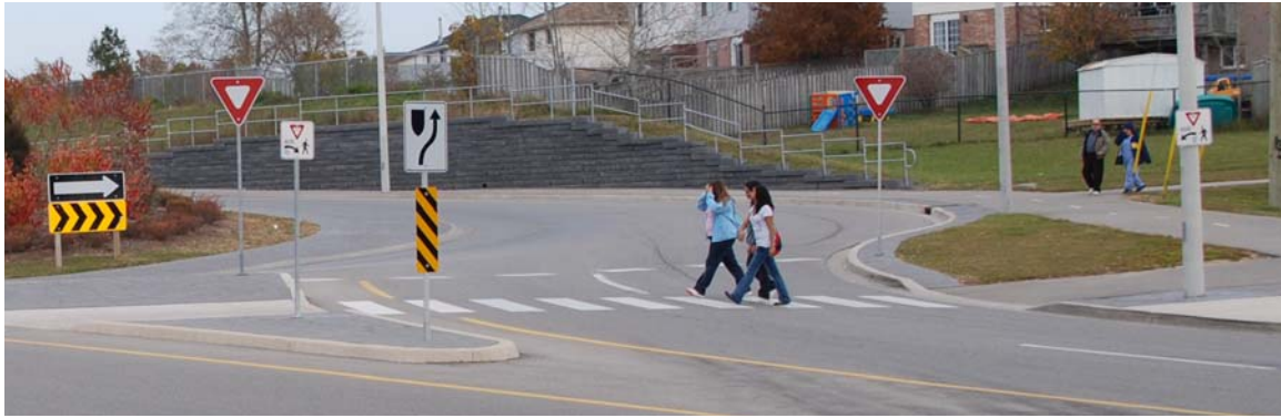
Figure 7 – Placement of “Yield to Pedestrians” Signs
