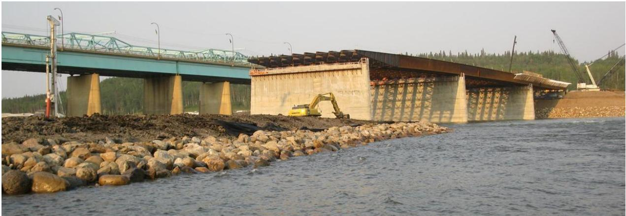
Figure 7. Incremental Launching of Steel Plate Girders for the Athabasca River Bridge
