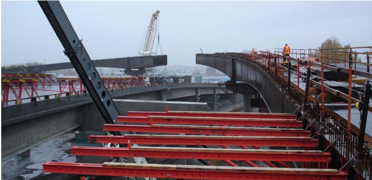
Figure 2. Progressive cantilever erection of the main-span over the railway lines and South Approach viaduct
