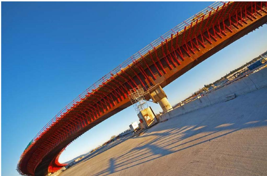
Figure 1. The Erected 199A steel box girder viaduct crossing the South Approach viaduct
