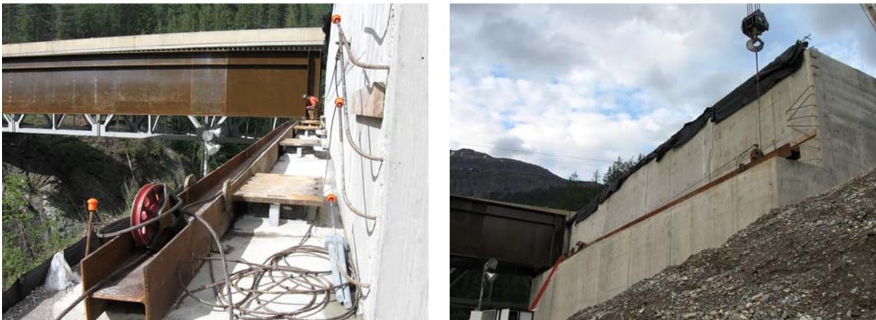
Figure 6. Installation of rigging (left) and lateral launch of girders (right) for the new Mount Hunter Creek Bridge
