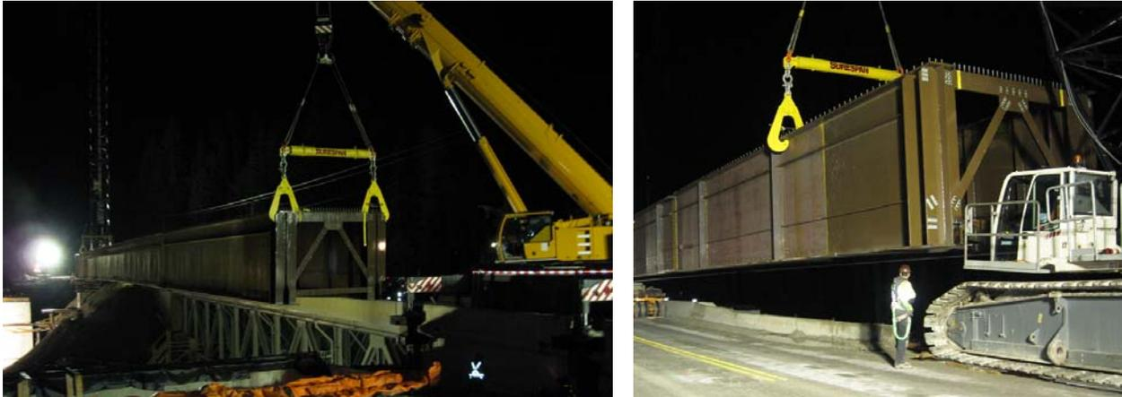
Figure 5. First critical lift for girder installation viewed from the west approach (left) and east approach (right)
