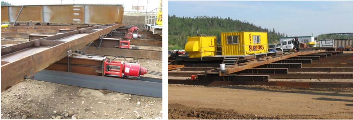
Figure 11. Sled beams, push beam, and strand jacks (left) and sea container housing launch equipment (right)
