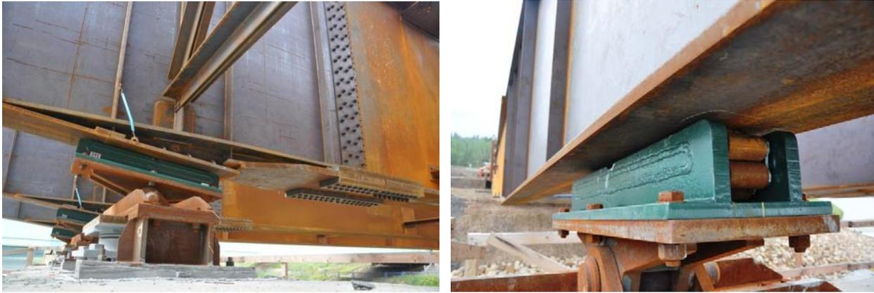
Figure 9. Launch nose (left) and girders (right) supported by a Hilman Roller during the launch
