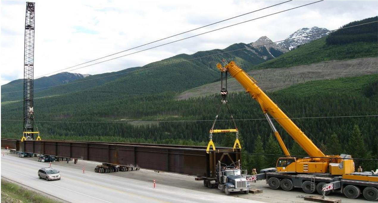
Figure 4. Two 300T cranes lifting a pair of girders onto dollies and a semi-tractor
