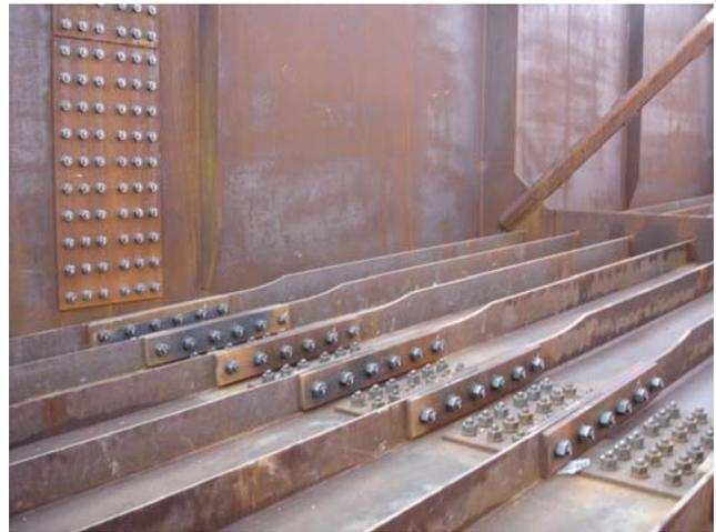
Figure 3. Bolting of a typical segment splice
