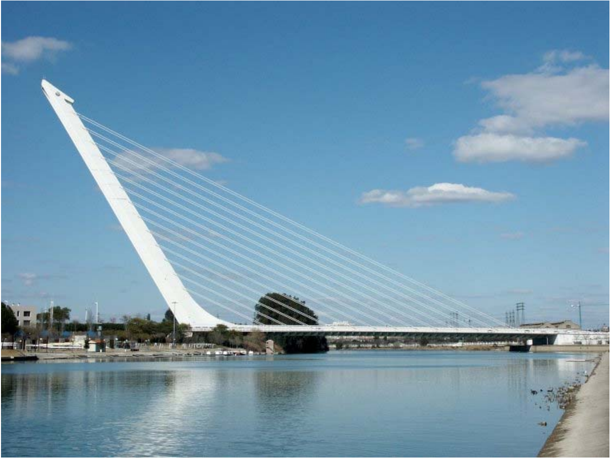
Figure 15: A Unique Structure Appears: Alamillo Bridge, Seville, Spain
