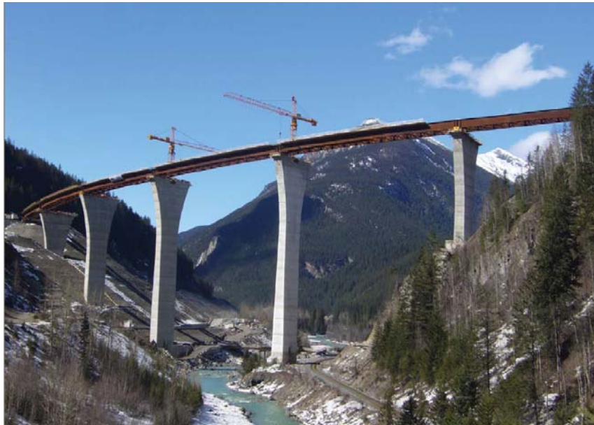
Figure 20: Kicking Horse Canyon Bridge, Kicking Horse, British Columbia
