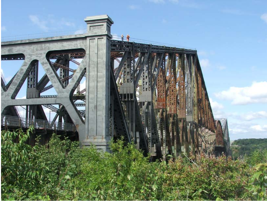
Figure 4: Quebec Bridge, Quebec
