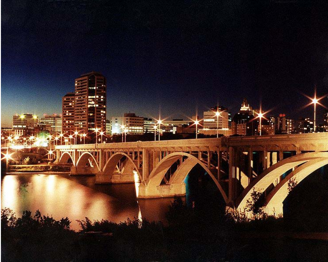
Figure 6: The Broadway Bridge, Saskatoon
