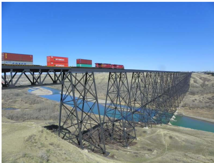
Figure 3: Lethbridge Viaduct, Alberta
