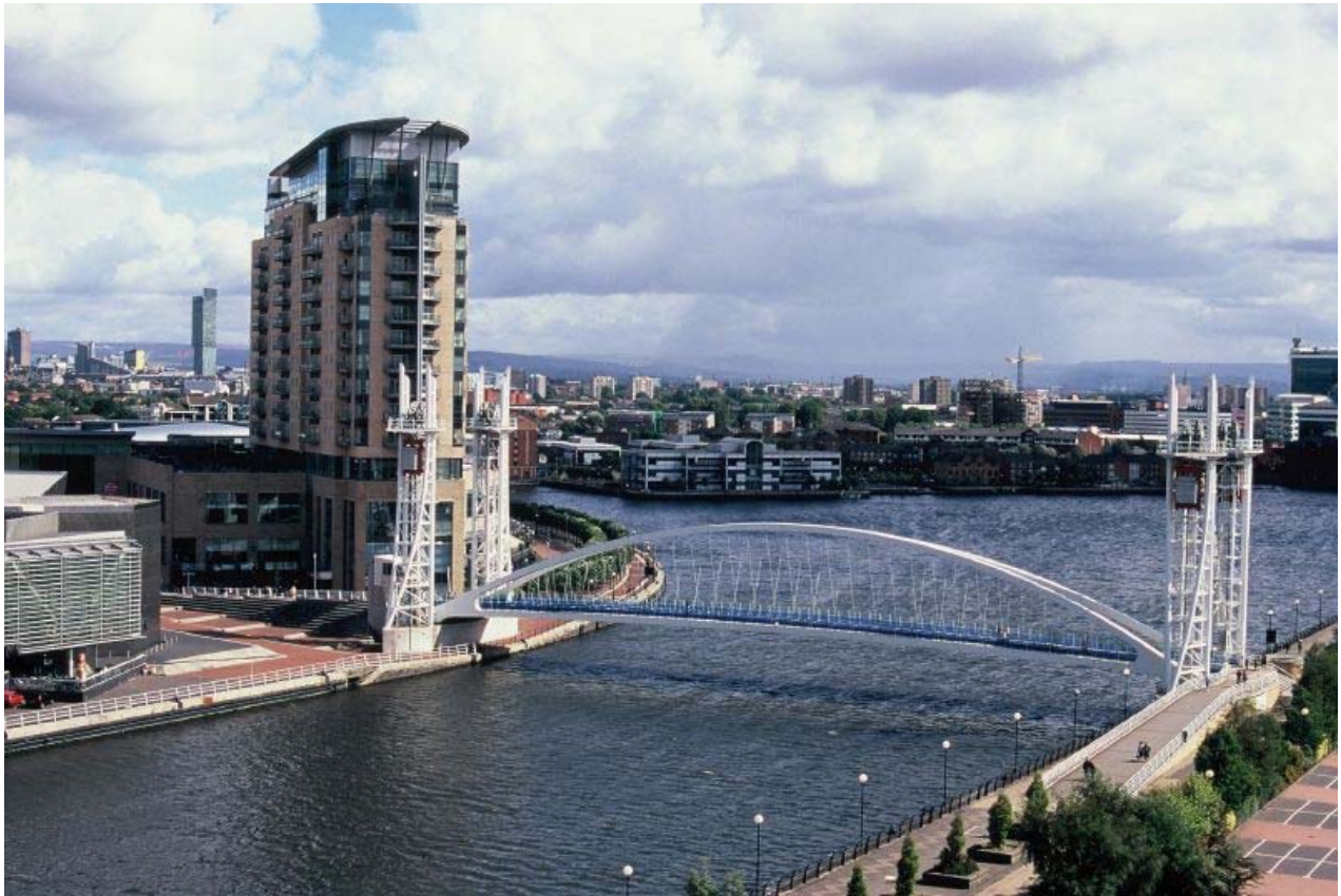
Figure 13: Lift Bridge at Salford Quays, Manchester, UK
