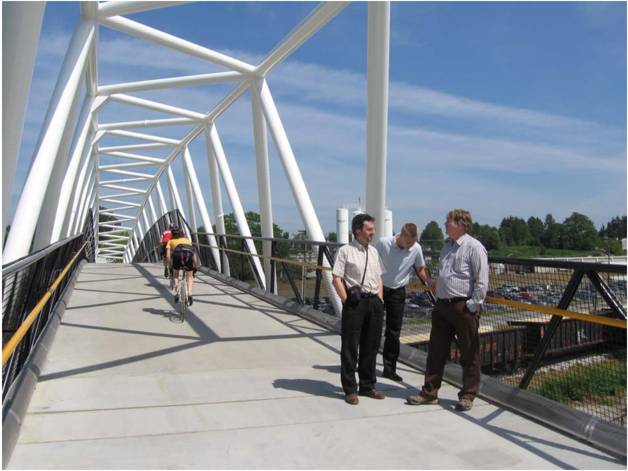
Figure 14: Winston Street Overpass, Burnaby, BC
