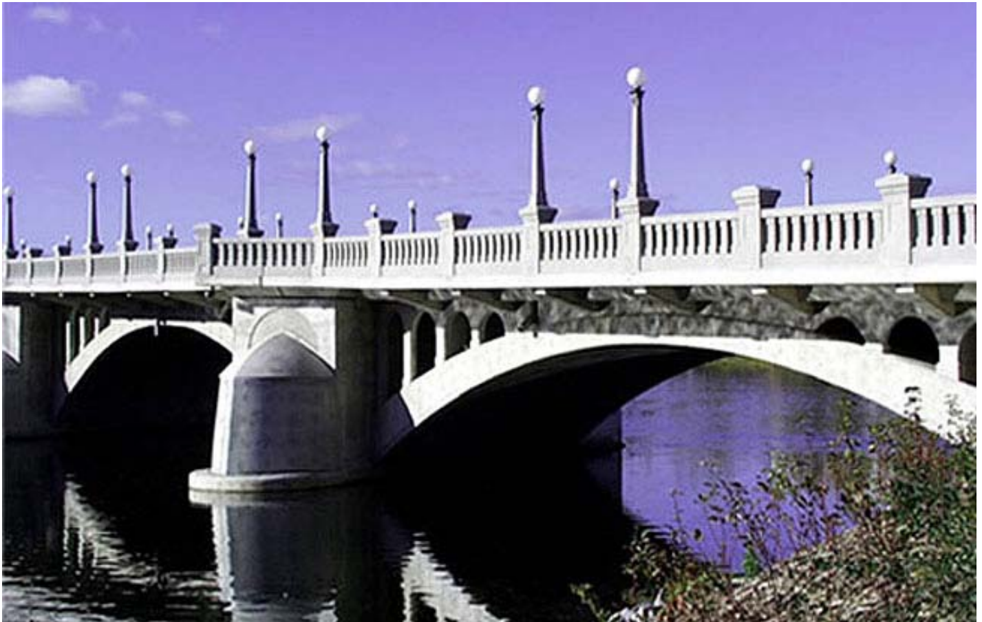
Figure 10: Cummings Bridge, Ottawa
