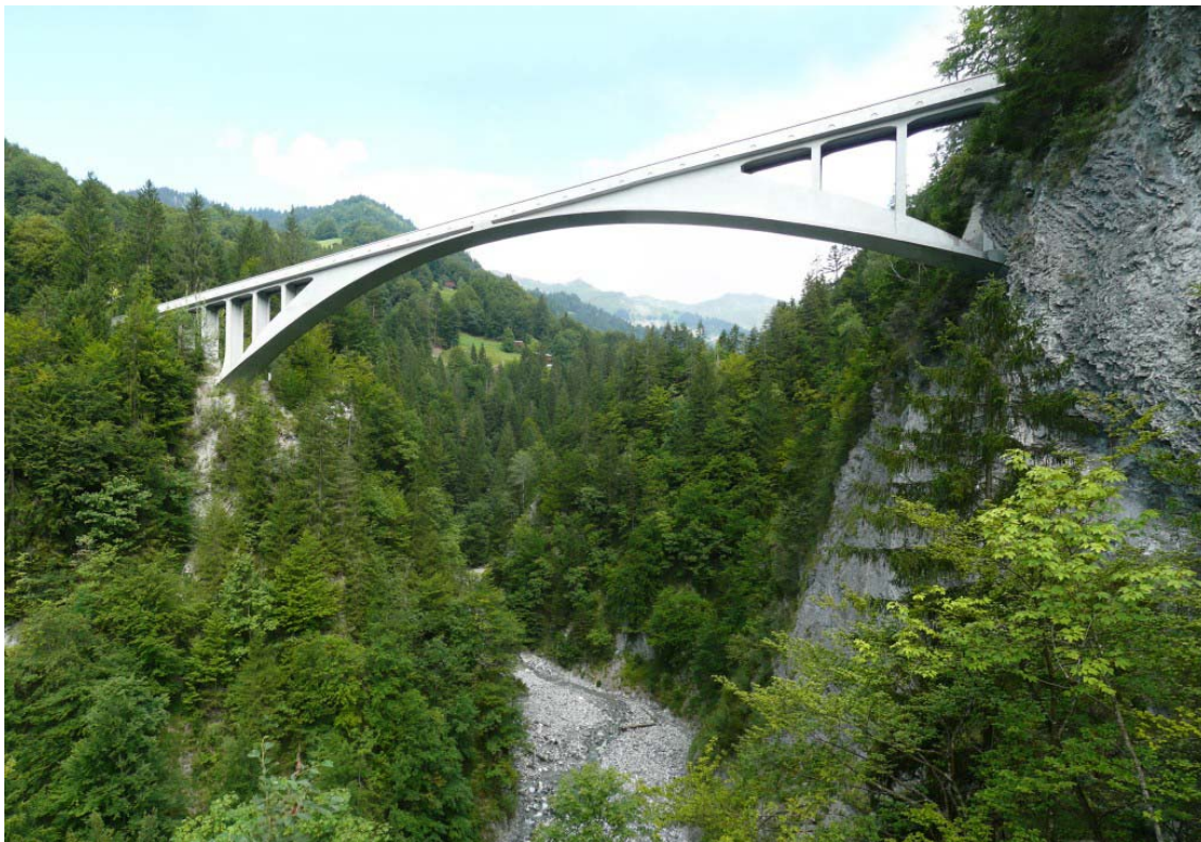
Figure 7: Salginatobel Bridge, Switzerland
