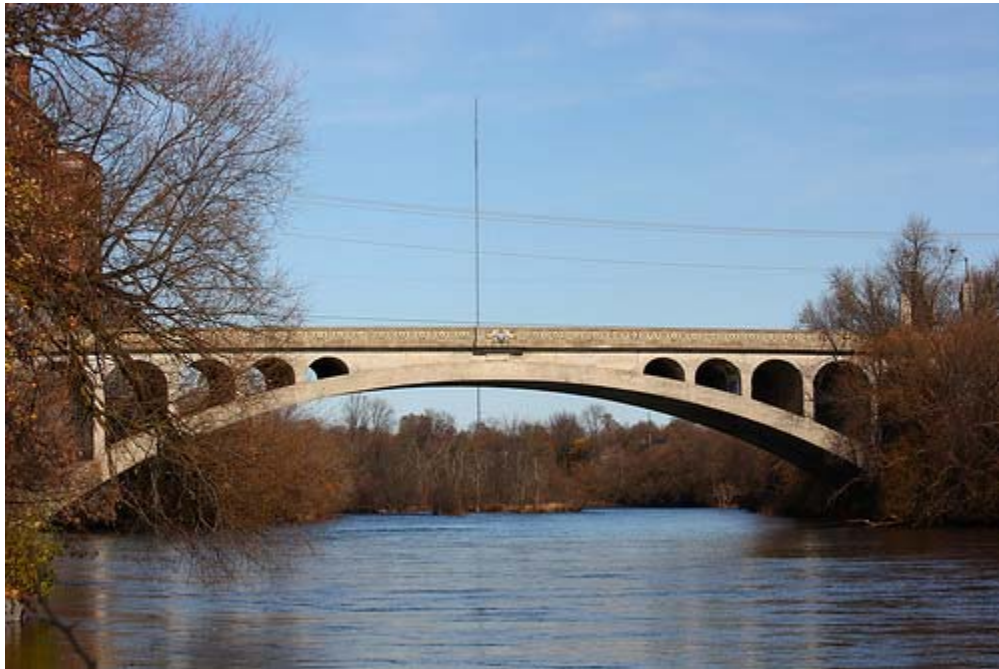
Figure 17: Hunter Street Bridge, Peterborough
