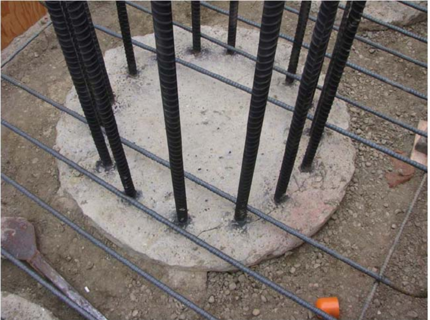
Figure 21 - Surface Cracks in Shafts
