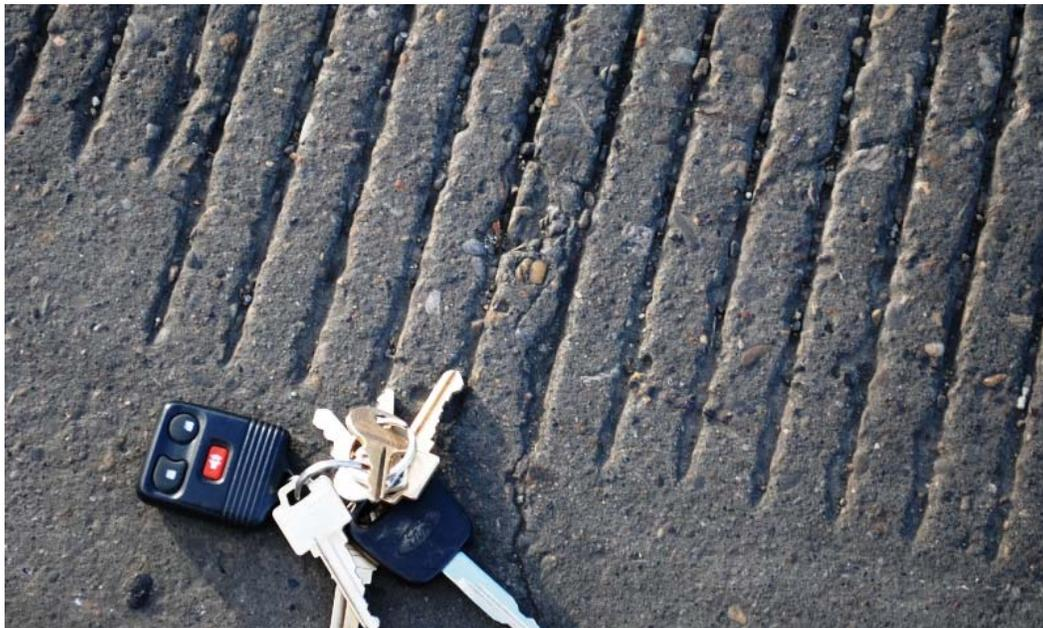
Photo 4: Map cracking and light surface scaling.
