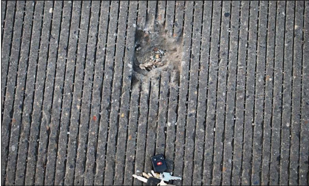
Photo 3: Spalling surface of the concrete overlay.
