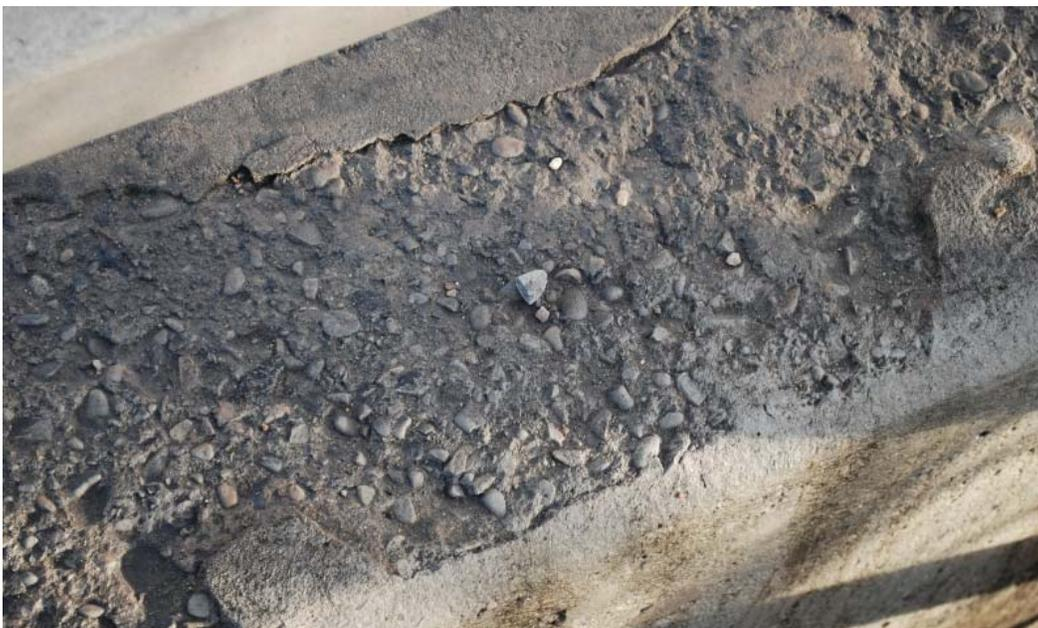
Photo 6: Spalling of concrete curb.
