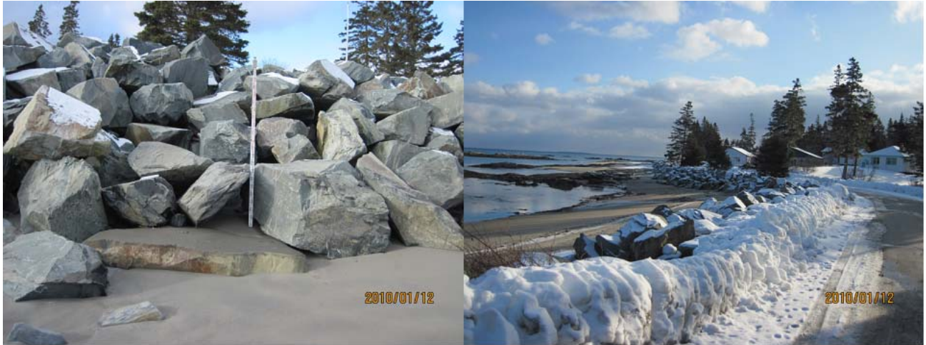
Figure 2 Ad hoc revetment at Green Bay, from beach and from road
