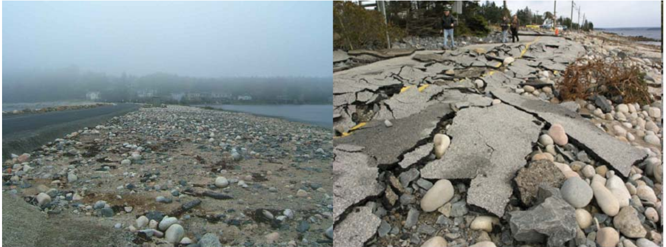
Figure 6. Damages to Queensland Beach roadway (Images courtesy NRCan 2007, NS Department of Fisheries and Aquaculture)
