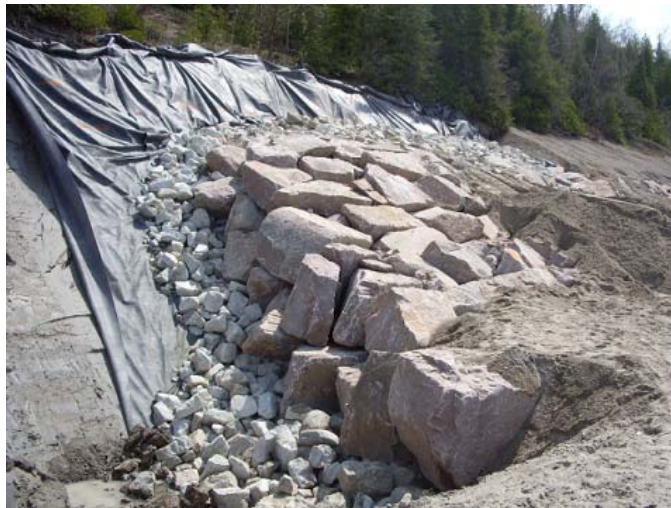
Figure 9. Example of an engineered two-layer revetment under construction
