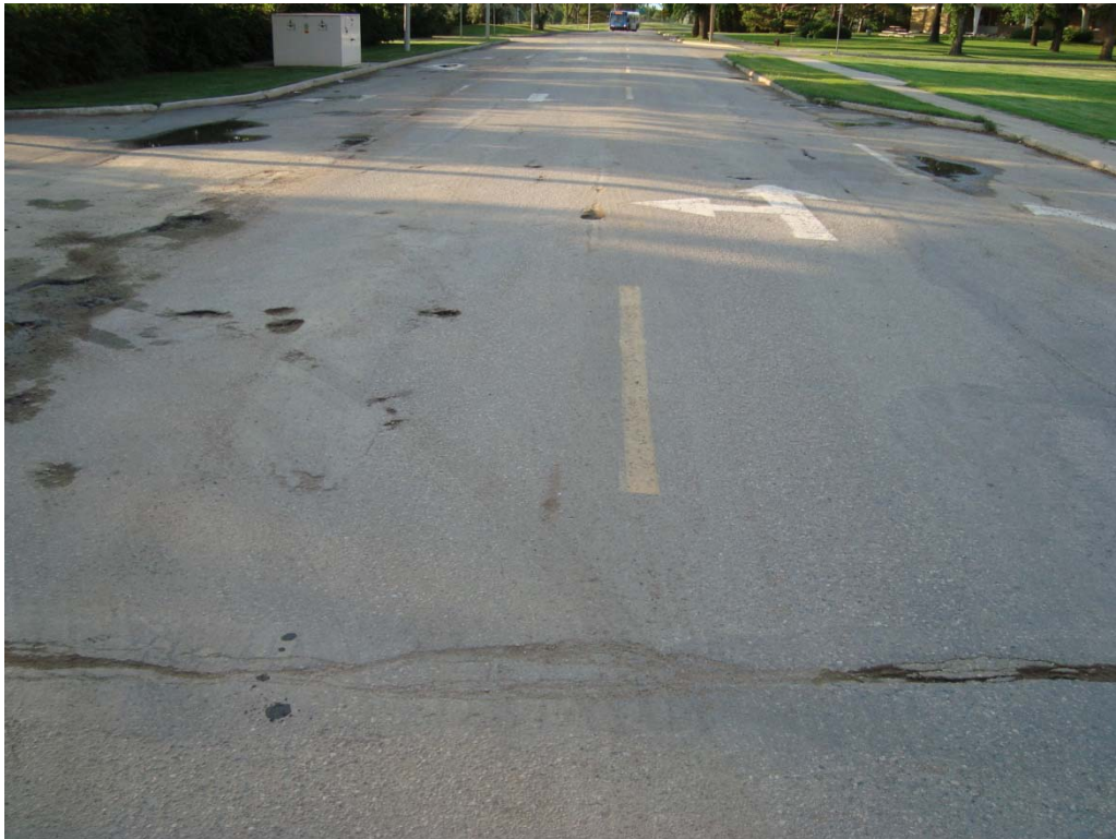
Figure 3 Typical surface distresses and structural failures of North Road – km 0.225
