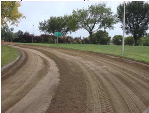
e) Preparation of reclaimed base layer
