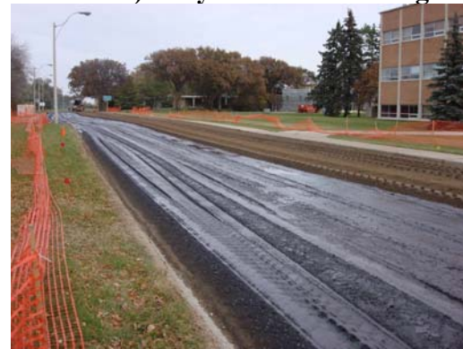
f) Engineered cold mix added
