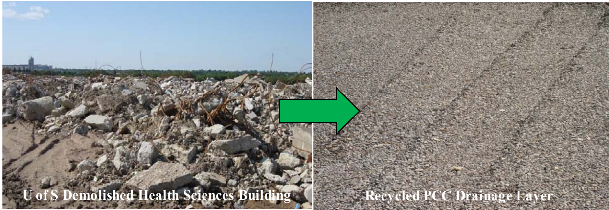
Figure 6 Rubble PCC Generated from U of S Demolished Buildings
