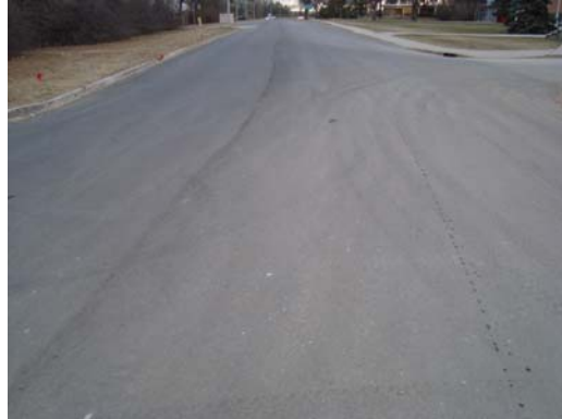
b) Section 2 engineered cold mix layer (left) and final HMAC surfacing (right)
