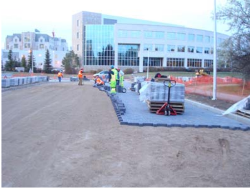
a) Section 1 sand bedding layer (left) and final paving stone surfacing (right)
