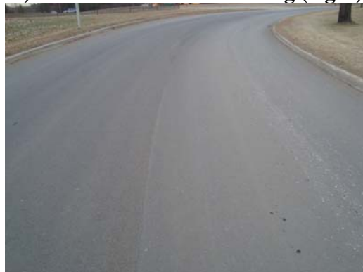
c) Section 3 stabilized reclaimed base layer (left) and HMAC surfacing (right)
