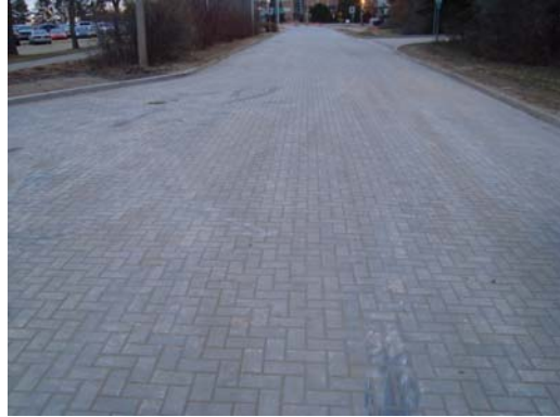
a) Section 1 sand bedding layer (left) and final paving stone surfacing (right)
