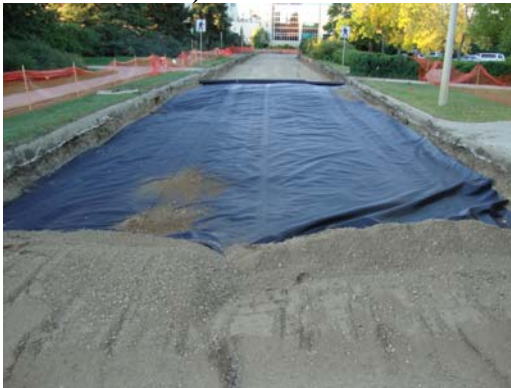
c) Installation of geotextile fabric
