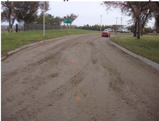
c) Section 3 stabilized reclaimed base layer (left) and HMAC surfacing (right)
