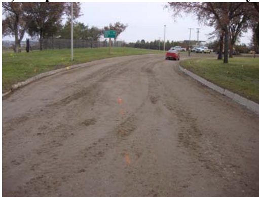
g) Base layer prepared for surfacing
