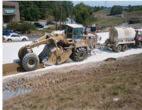
Figure 6 Self-powered rotary mixers blending host soil and hydraulic binders
