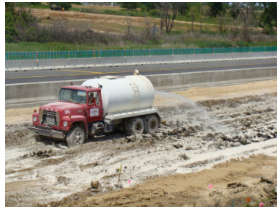
Figure 7 Water addition while mixing and/or directly after binder spreading
