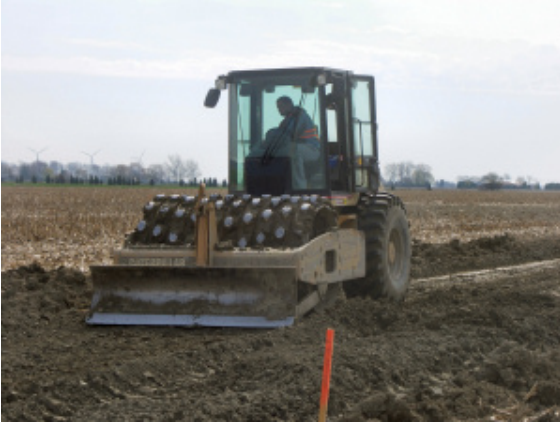
Figure 11 Initial compaction (pad foot) and the treatment train
