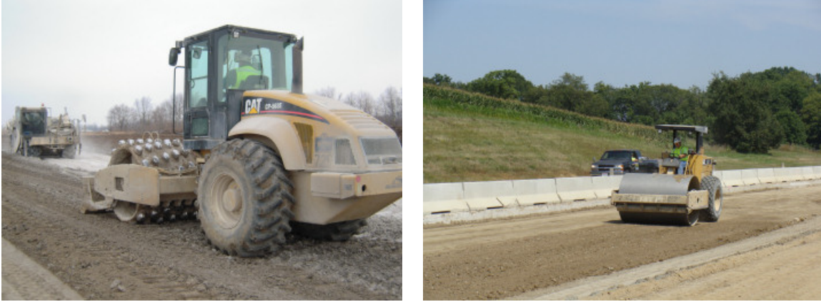
Figure 8 Initial compaction (pad foot) followed by final compaction (steel wheel)
