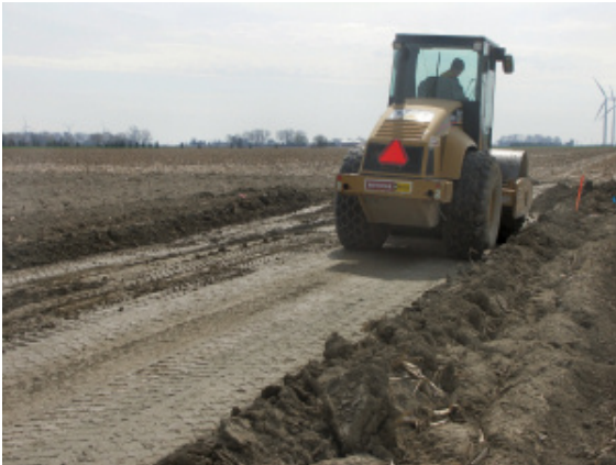
Figure 12 Final compaction and completed access road with granular surface
