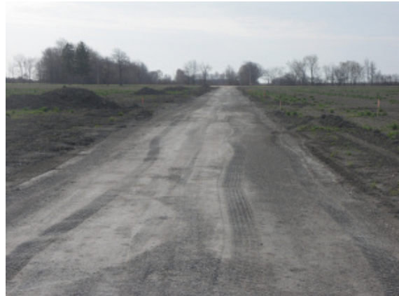
Figure 12 Final compaction and completed access road with granular surface
