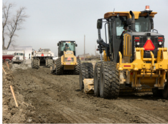
Figure 11 Initial compaction (pad foot) and the treatment train
