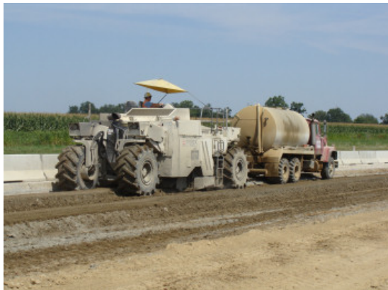
Figure 7 Water addition while mixing and/or directly after binder spreading
