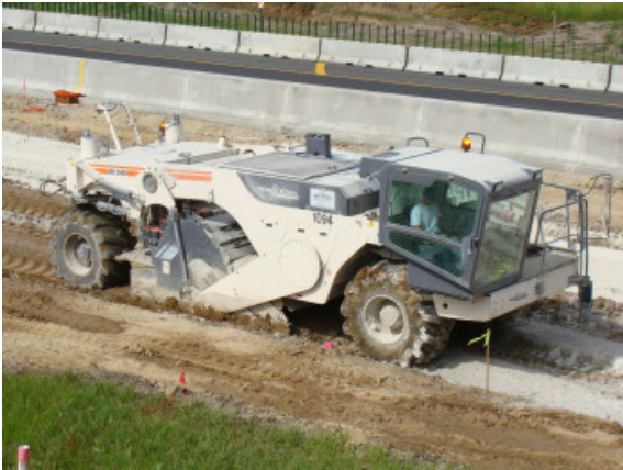
Figure 6 Self-powered rotary mixers blending host soil and hydraulic binders
