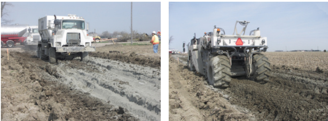
Figure 10 Site prior to treatment and processing binder into the natural soil
