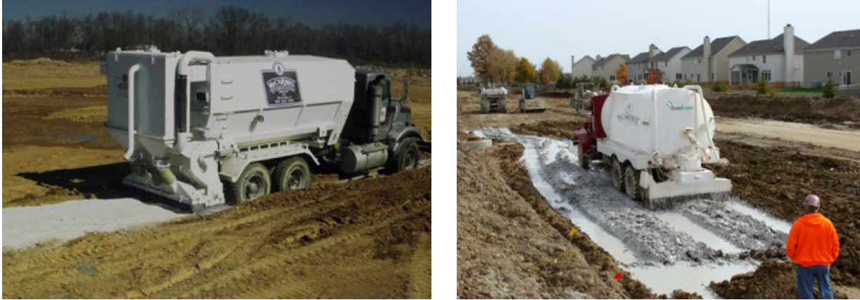
Figure 5 Spreading of hydraulic binder as a powder and as a slurry
