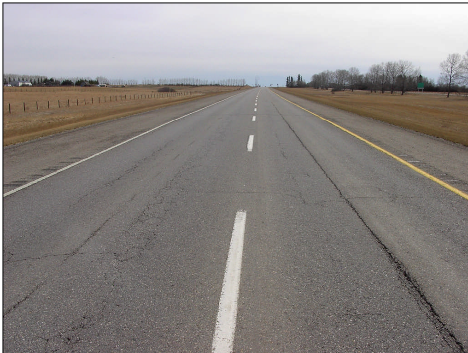
Figure 7. Typical Pavement Condition, Spruce Meadows Boulevard Westbound.
