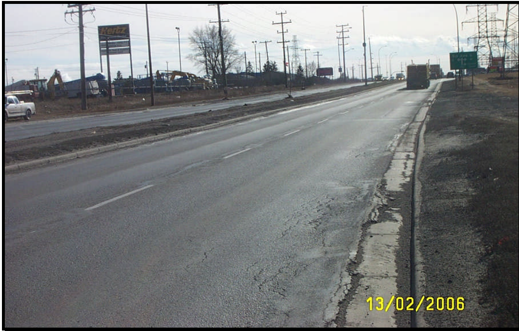
Figure 3. Barlow Trail, southbound lanes, between 50 Avenue and Peigan Trail, fatigue cracking in the outer wheel-path along curb lines, medium severity wheel-path rutting
