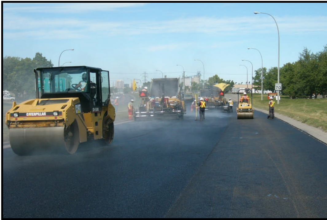
Figure 4. Barlow Trail Paving, northbound lanes, south of 61 Avenue.
