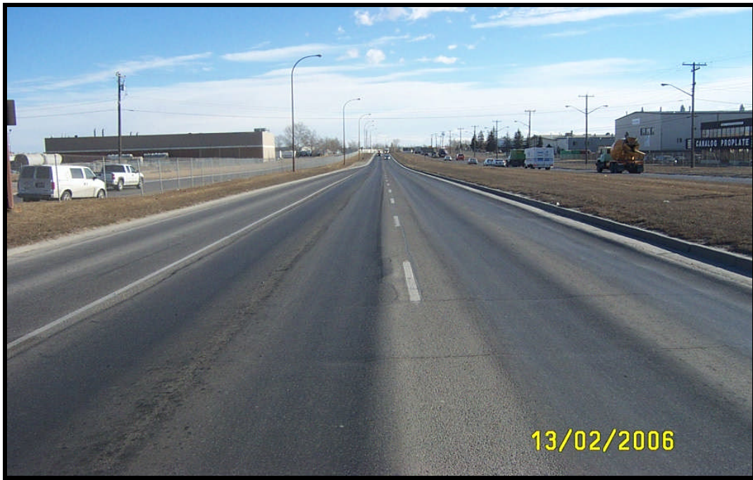
Figure 2. Barlow Trail, northbound lanes, between 61 Avenue and 50 Avenue, high severity wheel-path rutting.
