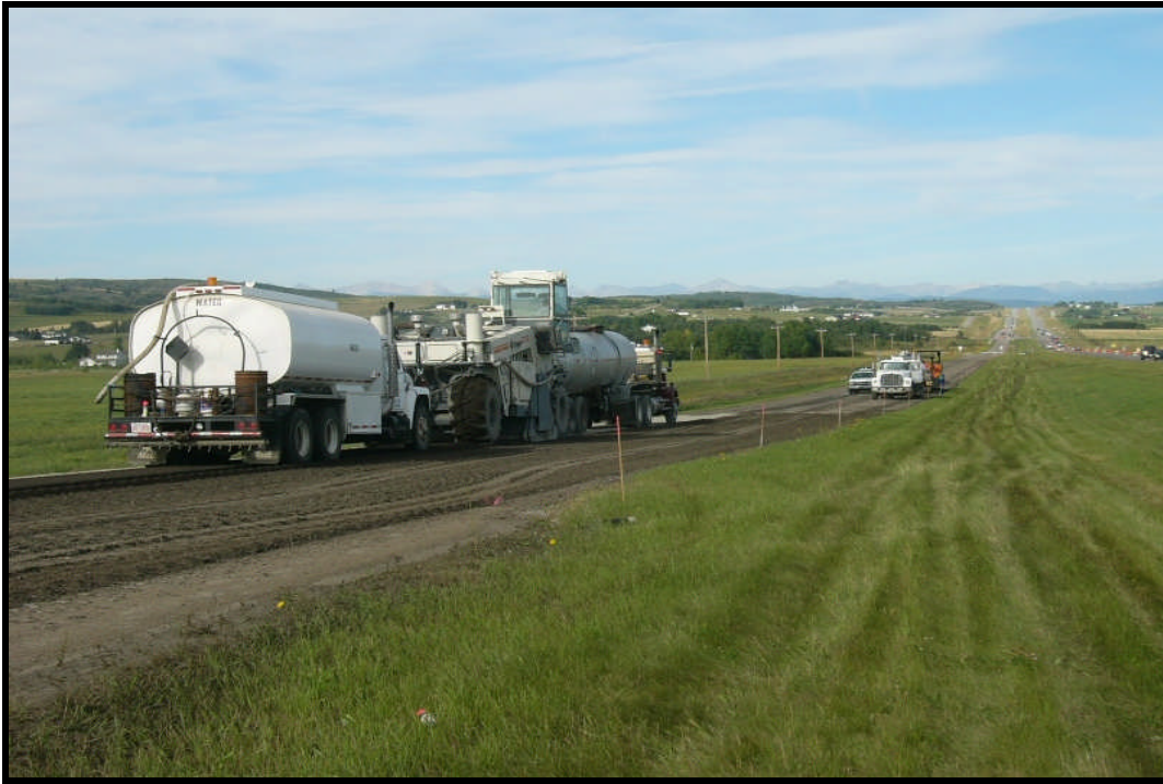
Figure 8. Spruce Meadows Boulevard Eastbound Lanes – FDR Construction
