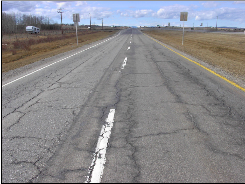
Figure 6. Typical Pavement Condition, Spruce Meadows Boulevard Eastbound.
