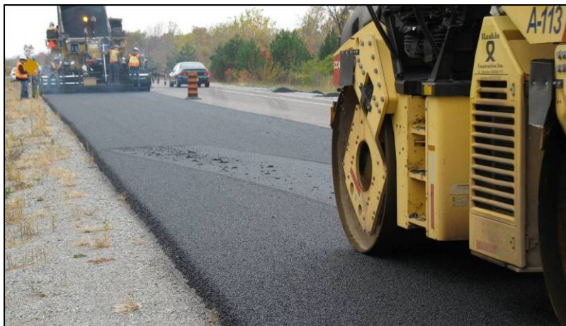
Figure 6 - Pick up of OFC asphalt mix during compaction
