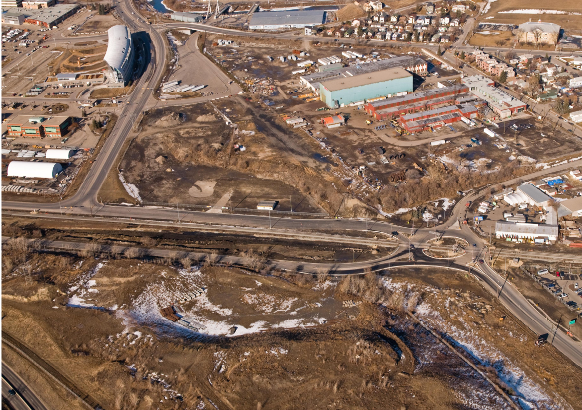
Figure 5 – Aerial Photography Showing Roundabout in Construction
