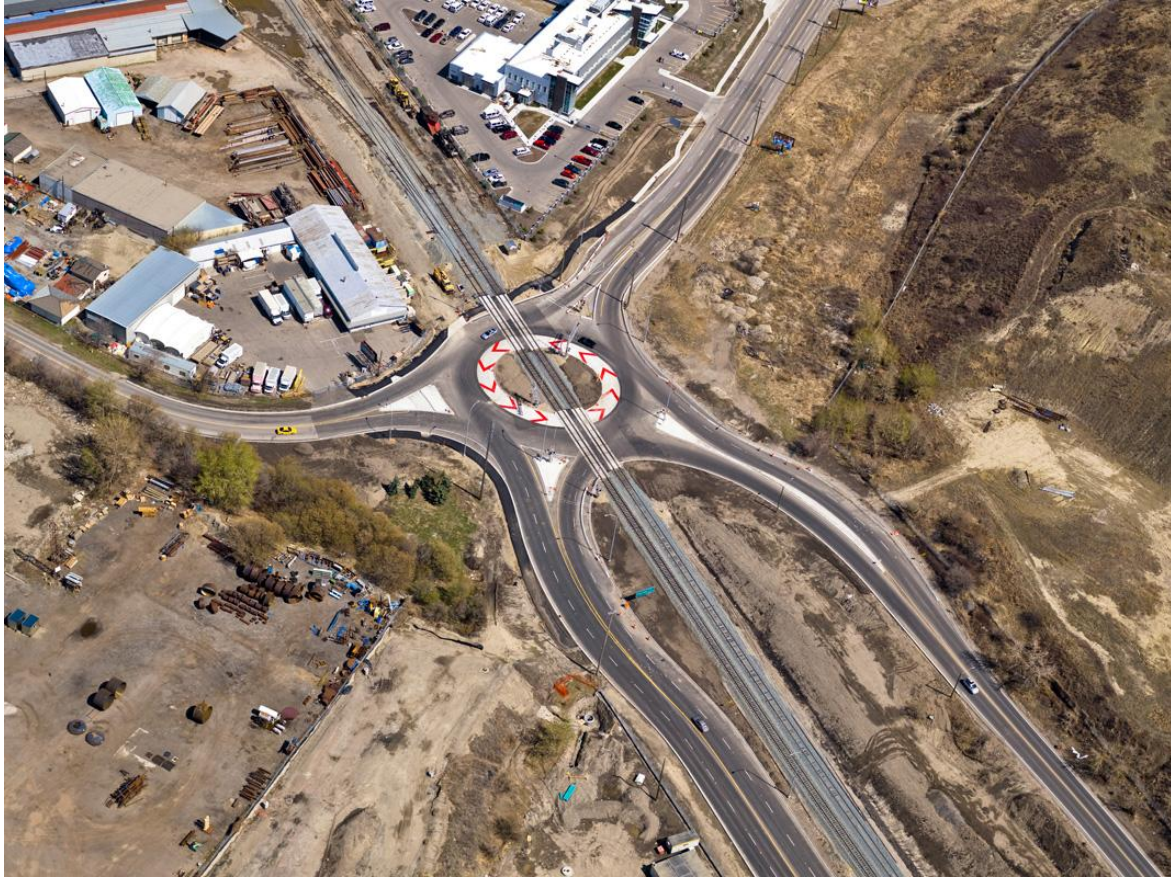
Figure 6 - Aerial Photography Showing Roundabout in Construction
