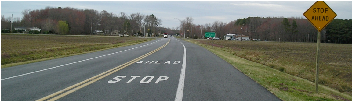
Figure 1: Example of a Rural STOP AHEAD Installation
