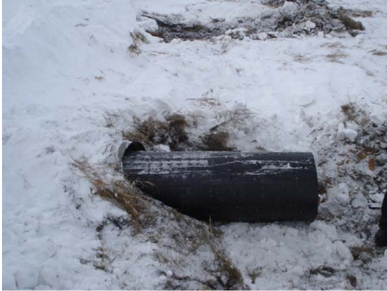
Figure 10 Installation of Snap-Tite® Liner at km 11.970
