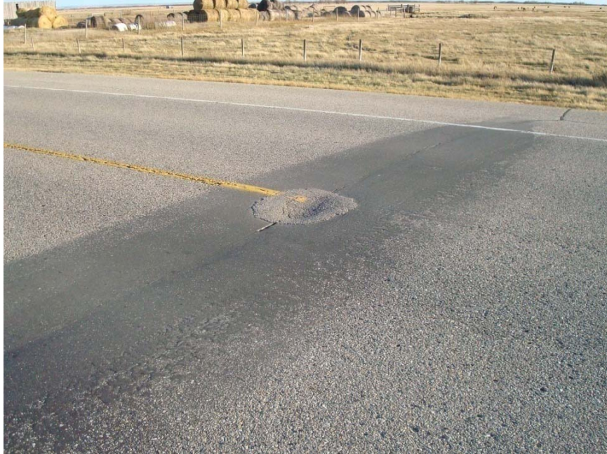
Figure 1 Surface cavitation as a result of culvert joint failure
