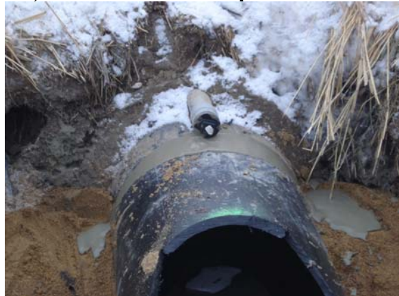
j) Culvert with Grouting Complete
