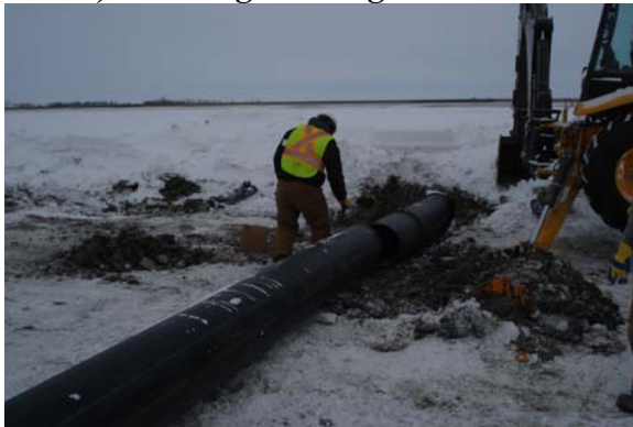
c) Insertion of HDPE Liner
