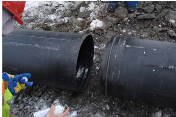
d) Aligning Sections of HDPE Liner
