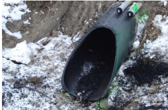
h) Trimmed End of Snap-Tite® Liner
