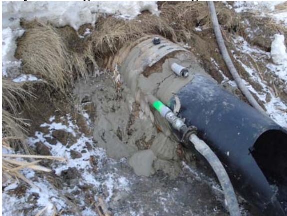
i) Grouting HDPE Liner into Place
