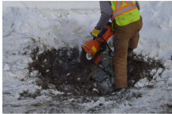
b) Removal of Damaged Culvert End
