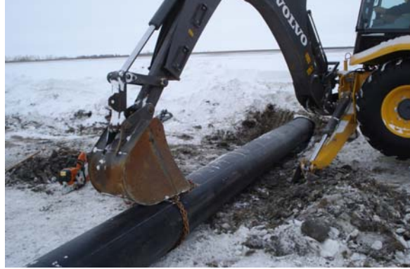
f) Insertion of Sections of Snap-Tite® Liner
