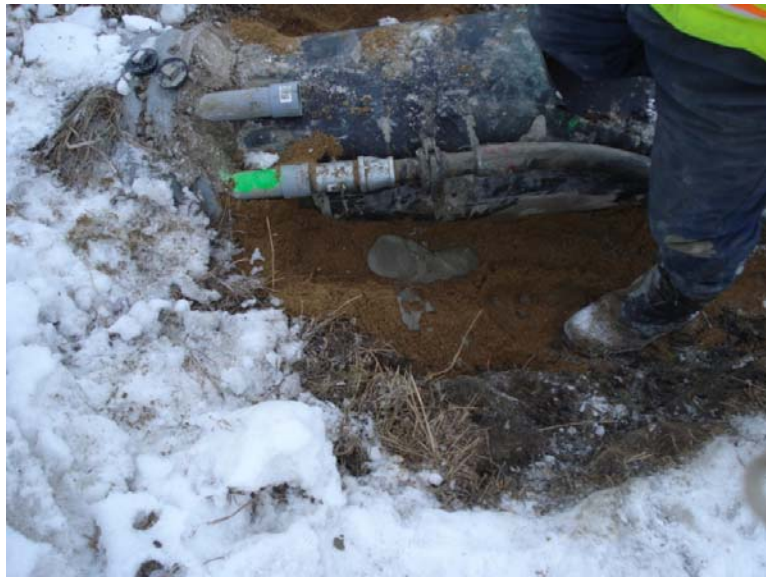
Figure 9 Grout Expelled Out of the Backfill at km 10.950
