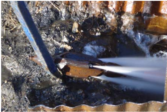
a) Cleaning Existing Culvert
