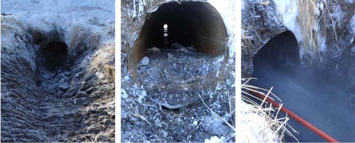
a) Culvert end submerged b) Culvert plugged with debris c) Cleaning culvert Figure 8 CSP Culvert at km 1.400
