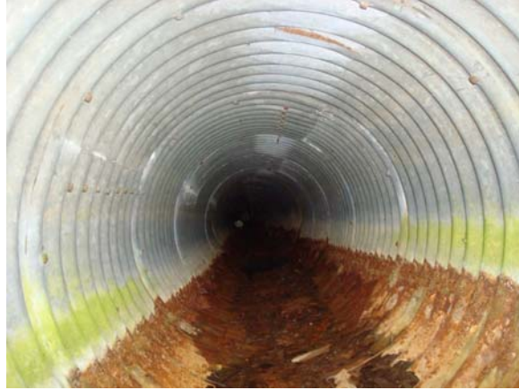
Figure 3 CSP culvert at km 10.950 (diameter of 600 mm)
