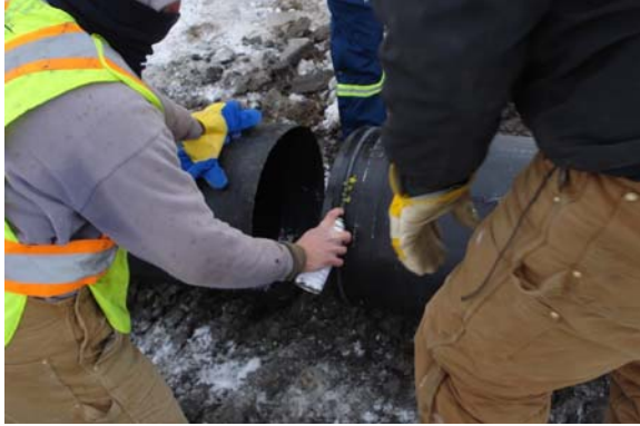
e) Lubricating of the Liner Joint and Gasket
