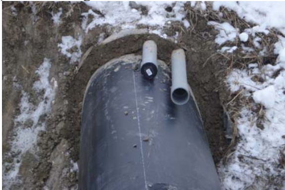
g) Dry Packing Ends/Installing Grout Tubes
