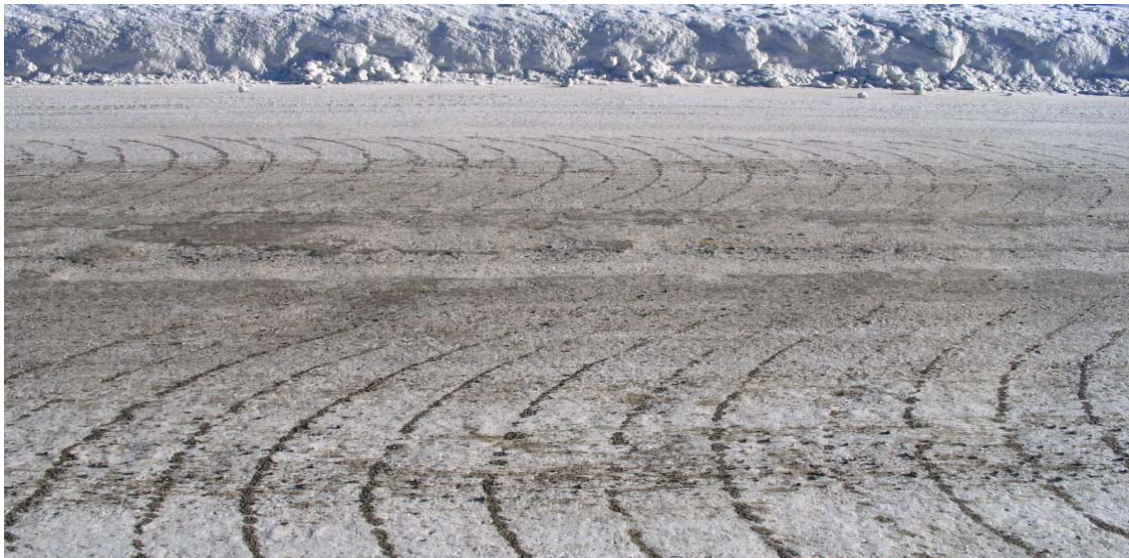
Figure 3: Arc spreading pattern on outbound and inbound lanes, Hwy 652
