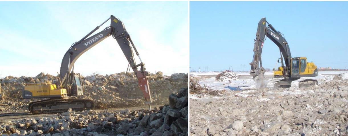
**Figure 5** PCC rubble processing: jackhammer (left) and muncher (right) (2009)
