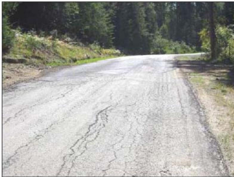
Figure 1 – Example of pavement distress indicating base problems.
