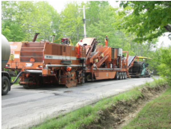
Figure 3 Trunk 8 PDR operations (left) and Route 236 FDR operations (right)
