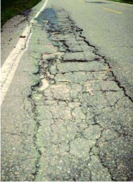
Figure 1 – Example of base failure cracking.
