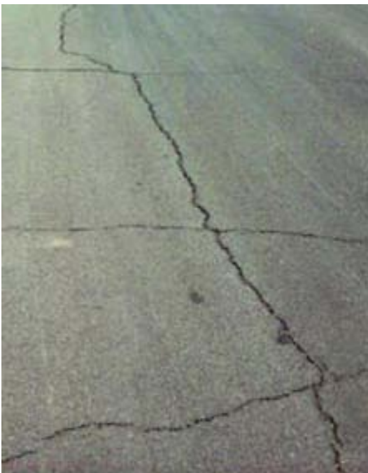
Figure 2 – Example of reflective cracking.
