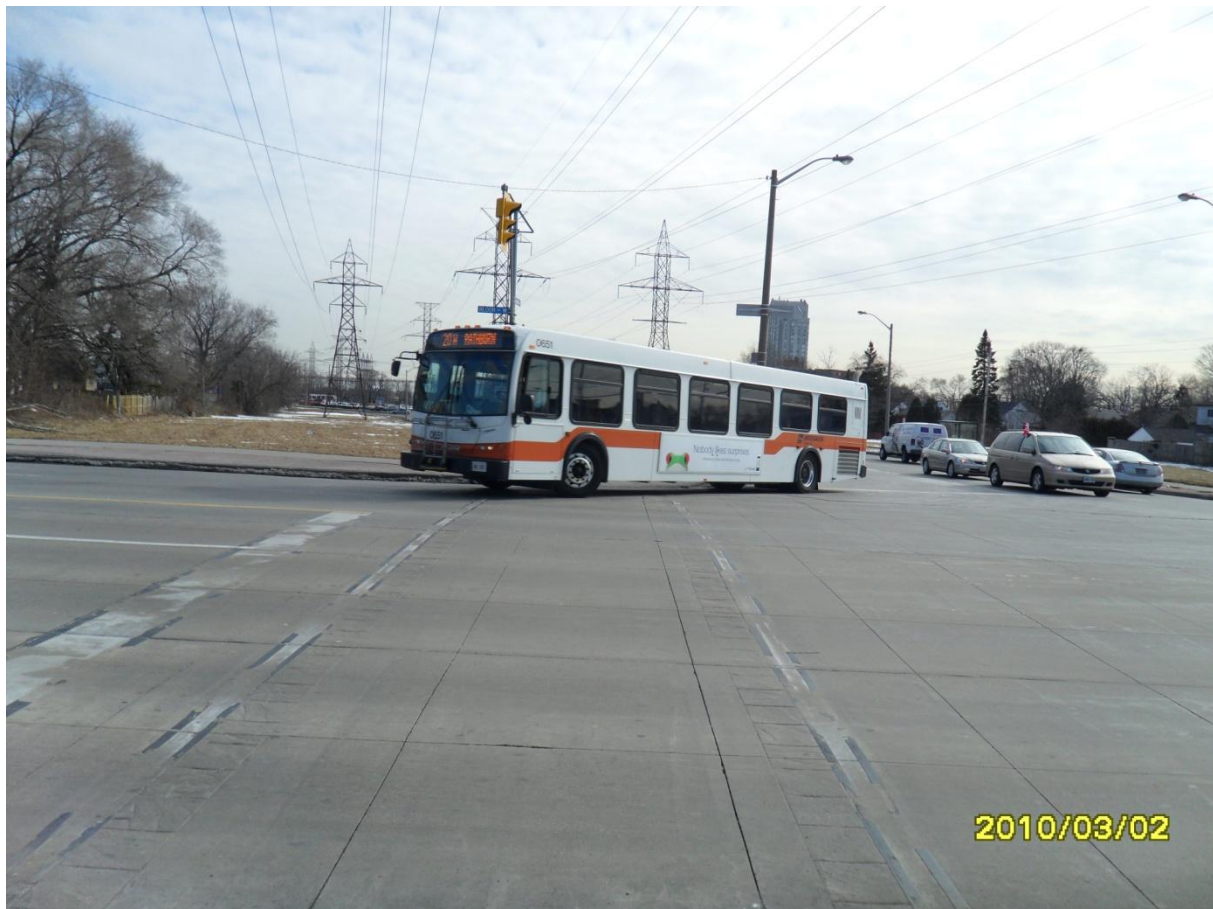
Figure 8: Bloor Street, Toronto Unbonded Concrete Overlay Condition after 6 ½ Years Service
