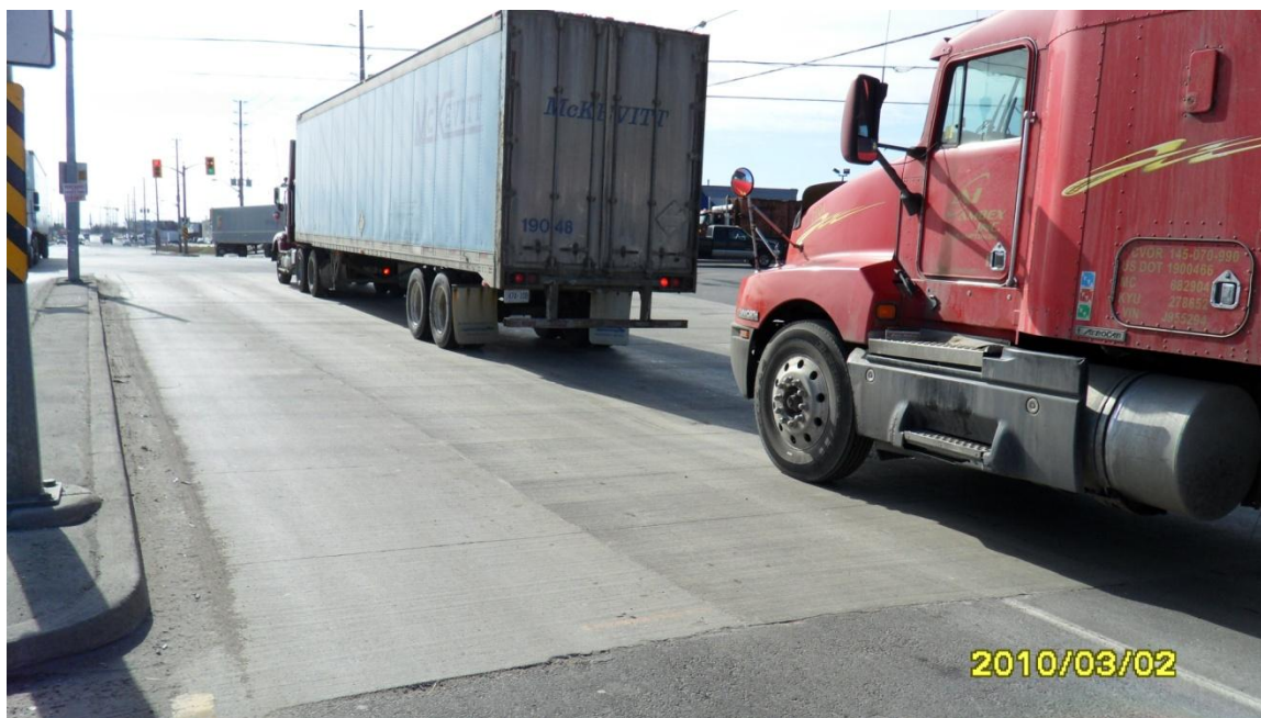
Figure 6 - Mississauga Bonded Concrete Overlay Condition after 14 1/2 Years of Service
